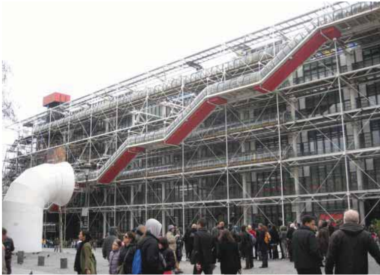
fig. 1.25 view of plaza and exterior escalator tube
