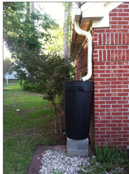
Figure 8. Rain barrel capturing roof runoff at a home in Horry County.
