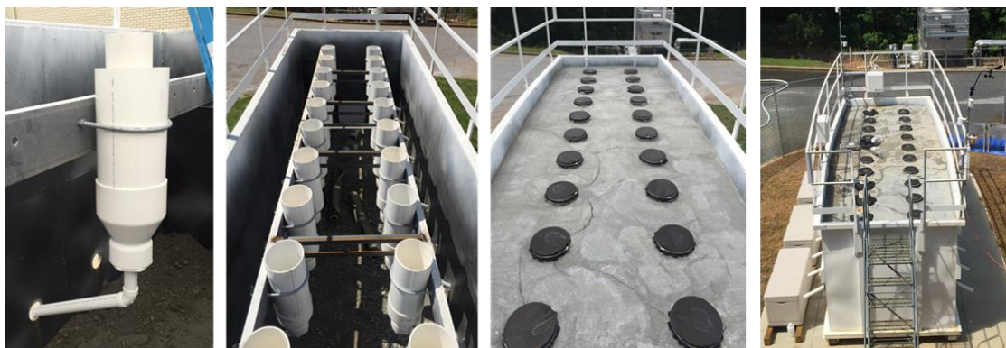
Figure 6.1: Lysimeter test bed construction showing the 20 outer casings.
