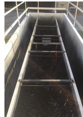
Figure 6.3: I-beam and angle iron placement.
