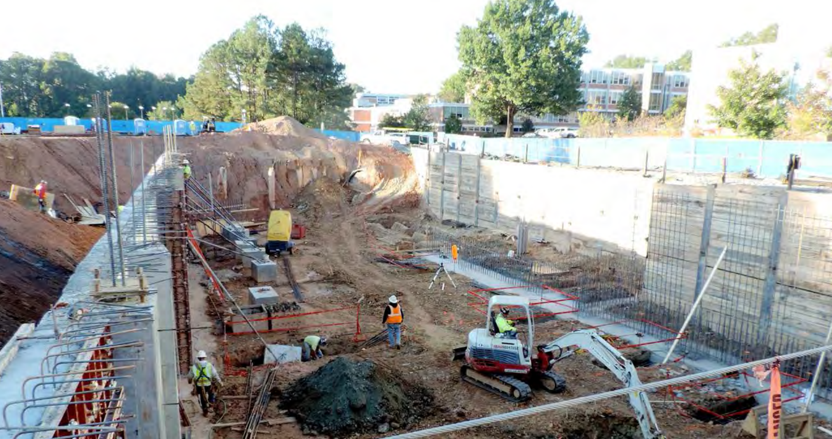
Foundation for the new Watt Family Innovation Center
