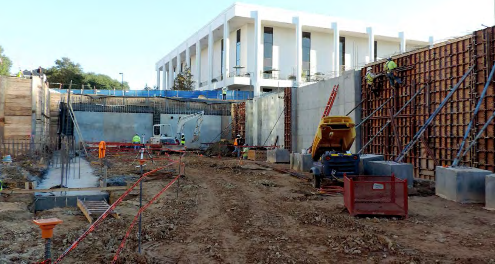
View of Cooper Library from Turner Construction site
