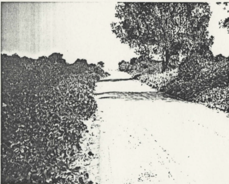
Erosion of road banks has been stabilized by kudzu on this road near Kelly, Union County
