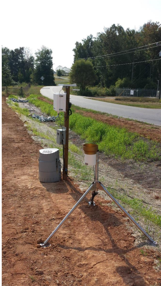
Figure 5.5: Instrument station and base station at bottom of the channel.
