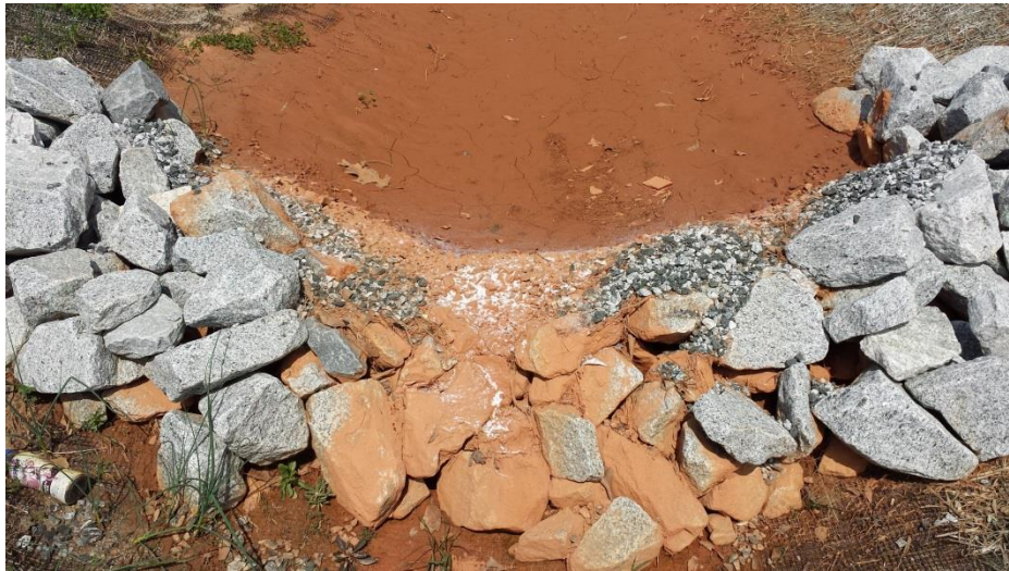
Figure 5.6: Rock ditch check with washed #57 stone on the upstream face and PAM.
