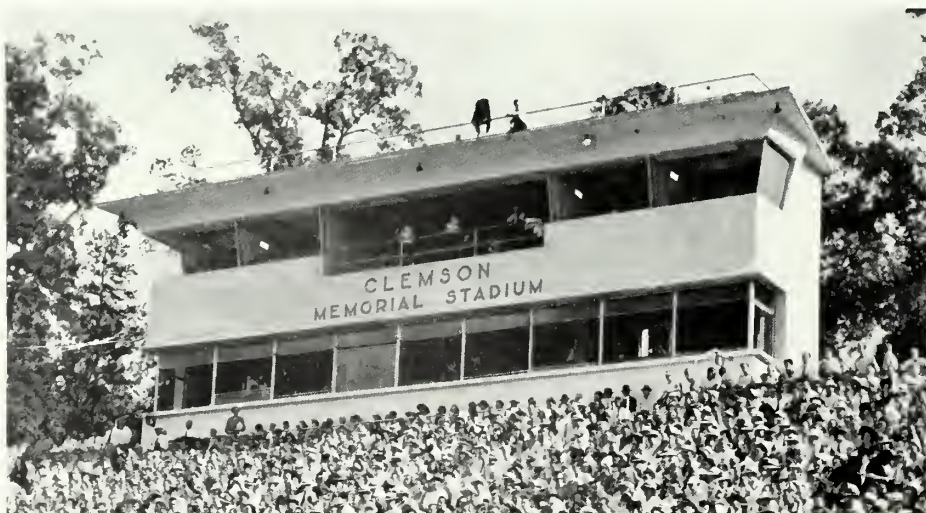
Bradley first worked in a press box reinforced by bamboo.
