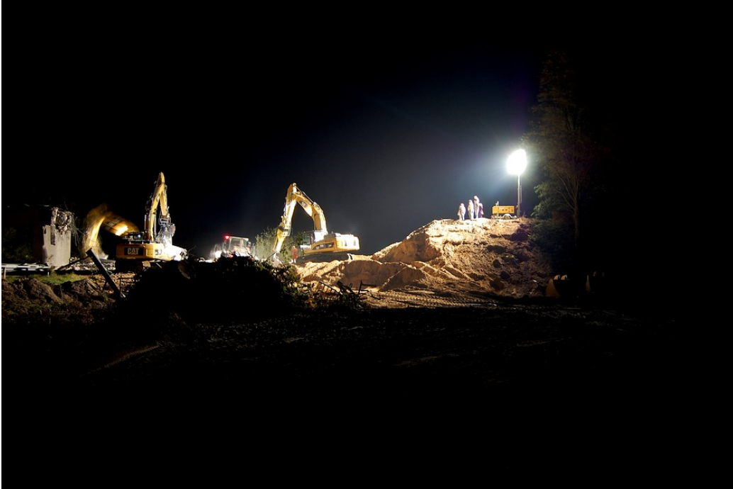
Figure 5.23: A single, bright spotlight aids the nighttime workers [22]
