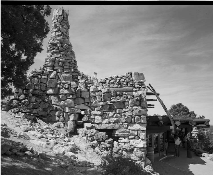
Figure 3.1 Examples of Parkitecture at Crater Lake (top) and Grand Canyon (bottom). Two different environments, yet easily identifiable as Parkitecture. Courtesy of the Library of Congress HABS Collection.
