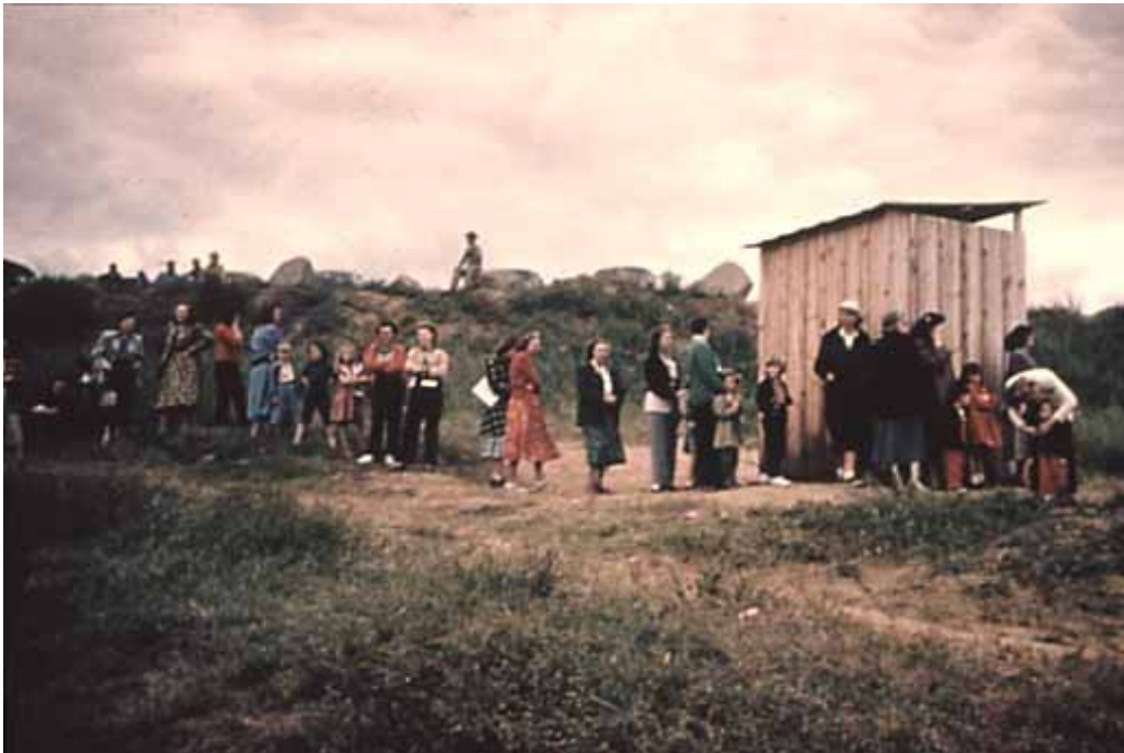
Figure 2.2 Outhouse line in a National Park, early 1950s. Allegedly when Director Wirth used this photograph in making his pitch for Mission 66 approval, this picture resonated the most with members of Congress. Courtesy of Historic Photos Collection: Harpers Ferry Center, National Park Service.
