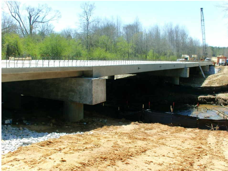
Figure 4: Hanging Rock Creek Bridge
