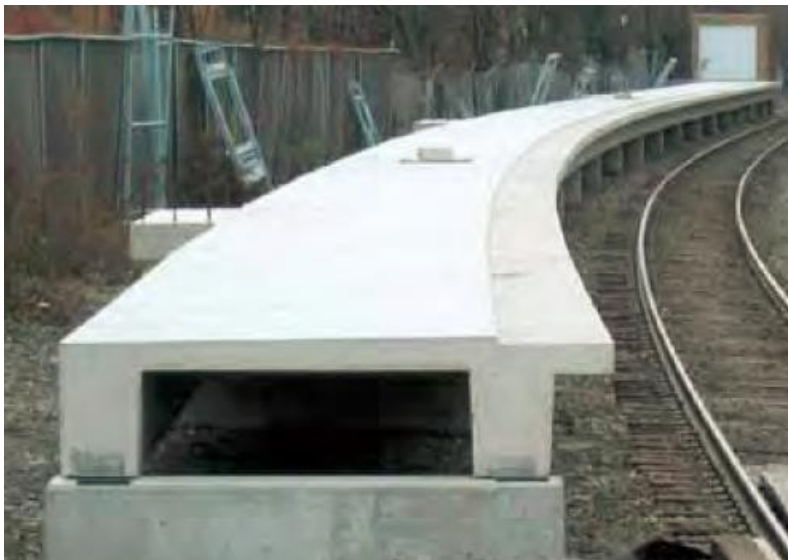
Figure 15: High-Level Railroad Platform that Inspired NEXT Beam Design (Culmo and Seraderian, 2010)
