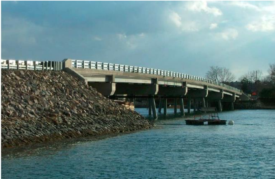
Figure 53: The New Bridge in York, ME (Gardner and Hodgdon, 2013)
