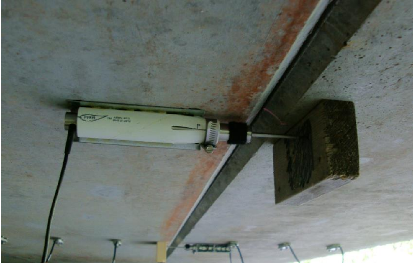
Figure 89: LVDT Mounted to Solid Slab
