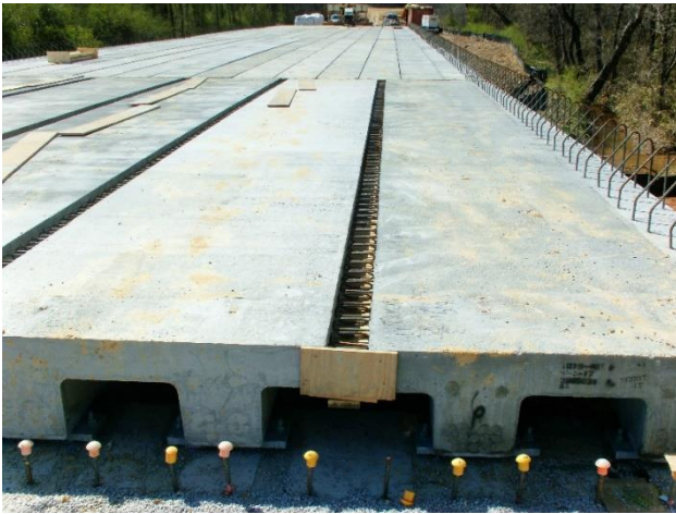
Figure 5: NEXT D Shear Key
