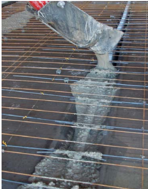
Figure 16. Concrete placement in stem
