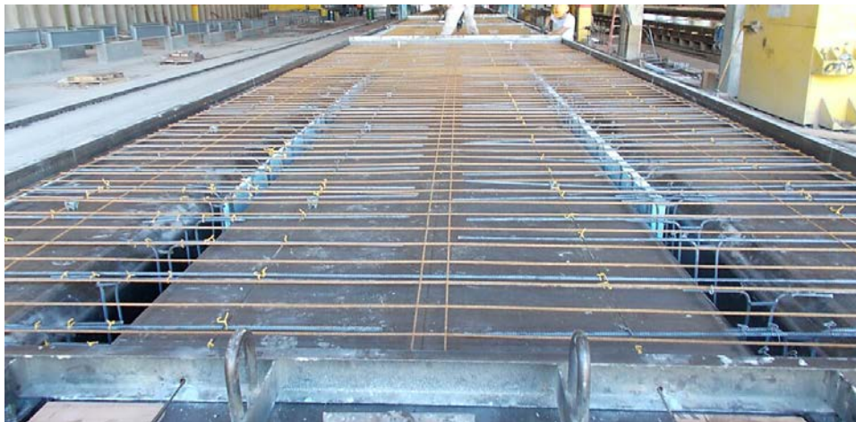
Figure 15. FVDT prior to casting
