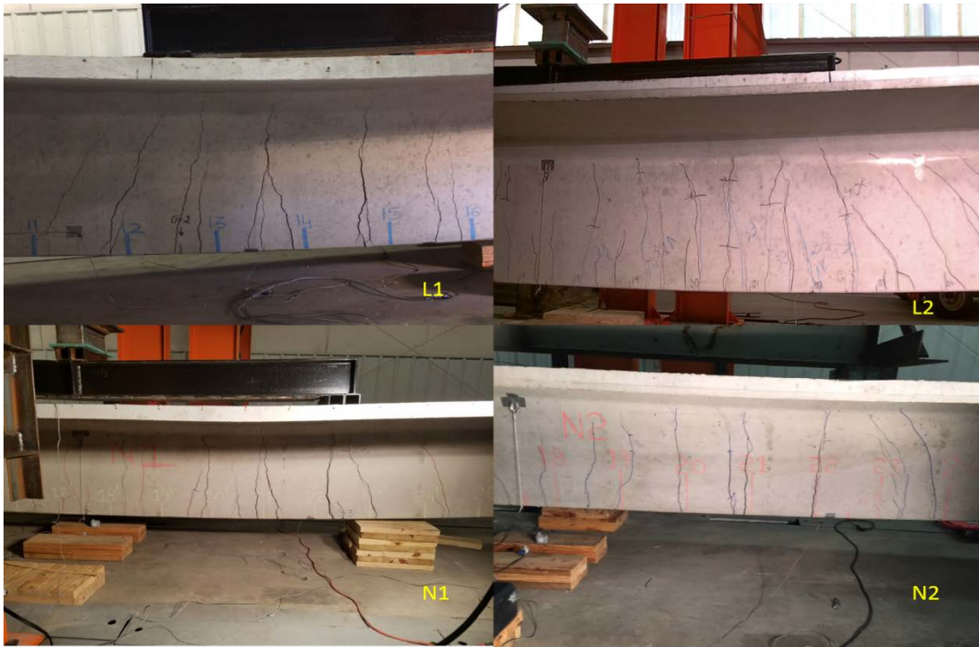
Figure 33: Crack pattern around mid-span of all the beams during flexural load test
