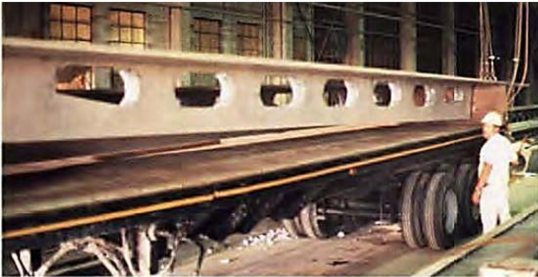
Figure 6. Single tee with web openings (photo courtesy- M. Tadros)
