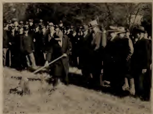
DOCTOR SIKES breaks ground, thus the textile building was begun
