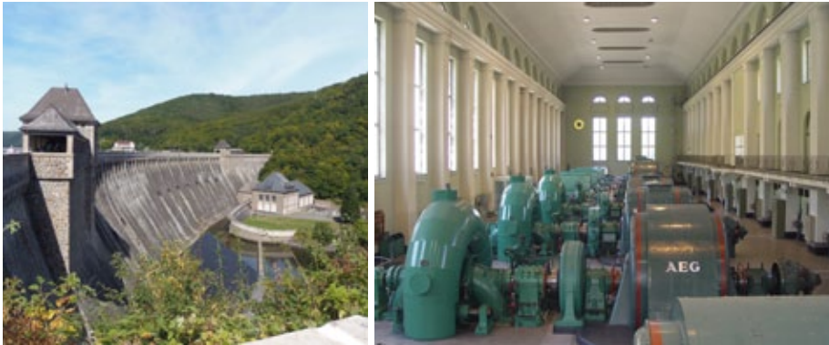
Figure 11 (l.): Edersee Dam, 2012 (By SJB1120, CC-BY-SA-3.0 via Wikimedia Commons)
