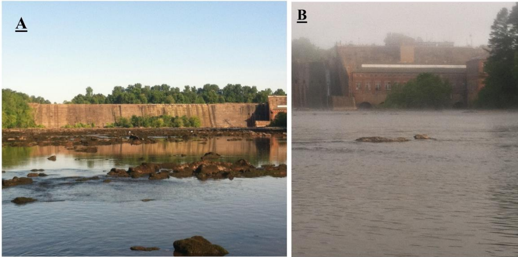
Figure 3-5. Photos of the Ninety-Nine Islands tailrace during low discharge (A) and high discharge (B) conditions.
