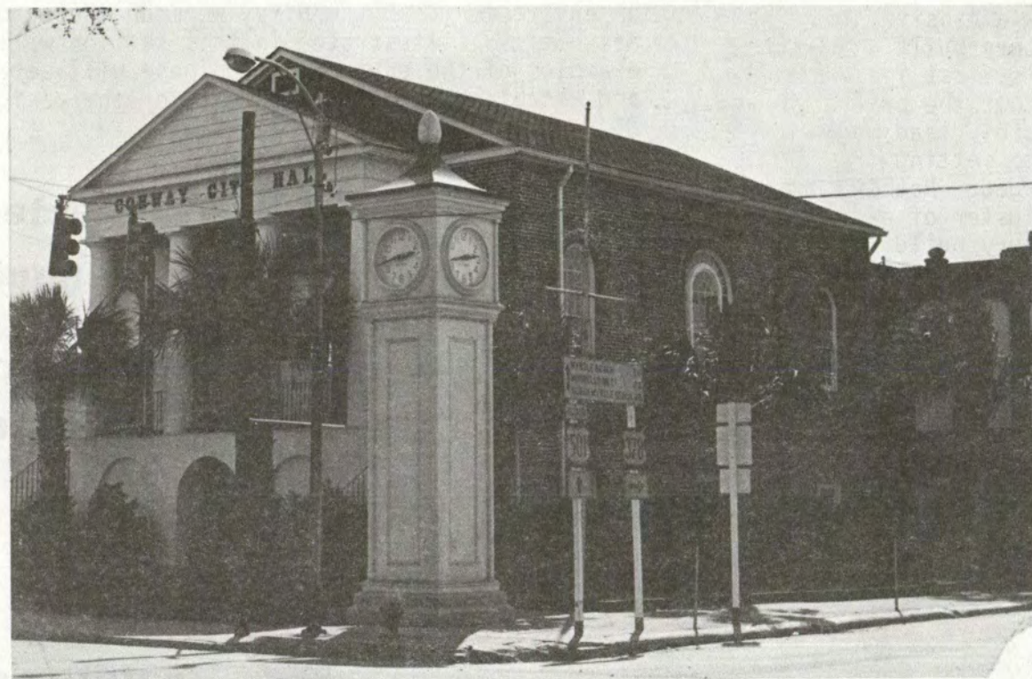
This building, constructed of brick with vaulted record rooms of massive arched masonry, was erected in 1824-1825 as a courthouse for Horry County. It is a typical Mills' design, having been erected under the administration of Robert Mills, then Commissioner of Public Works.
