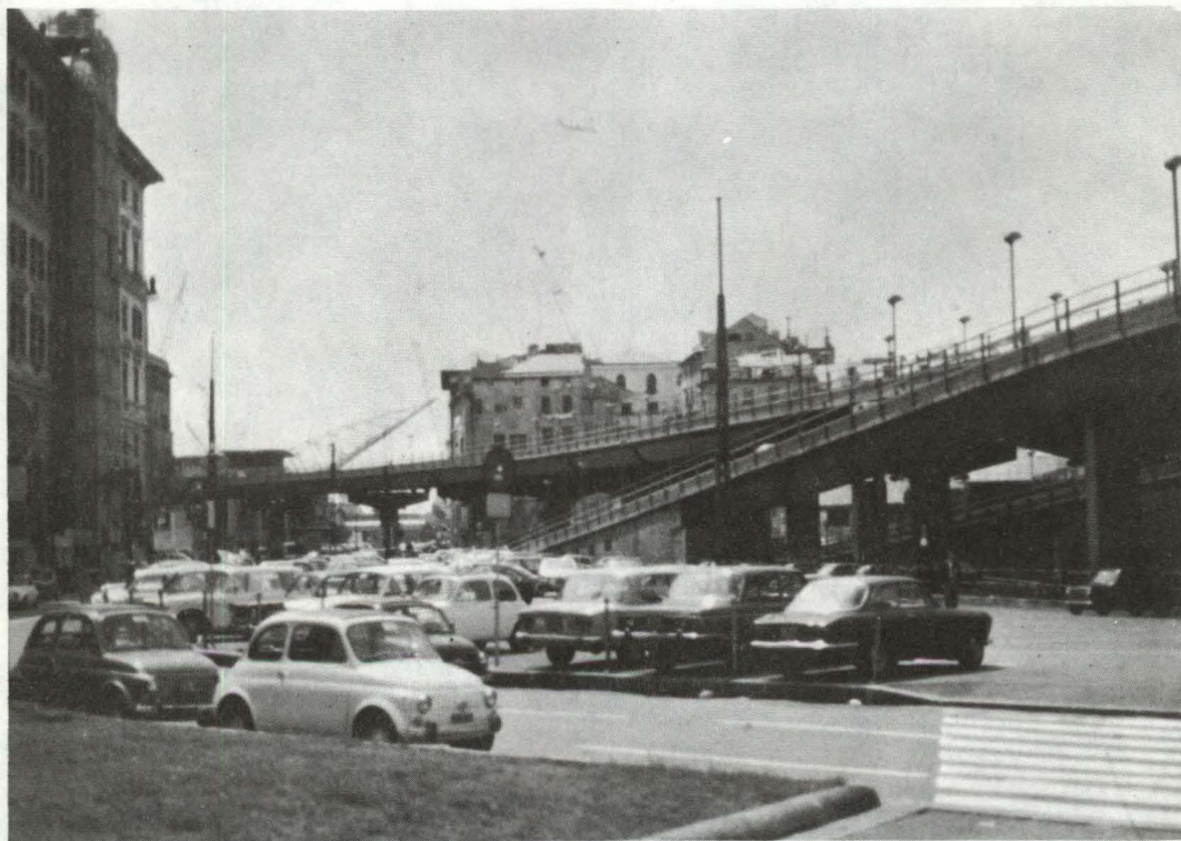
The elevated roadway is a strong psychological and visual barrier which separates the jetty from the city. The buildings behind the roadway are some of the residences on Molo Vecchio.
