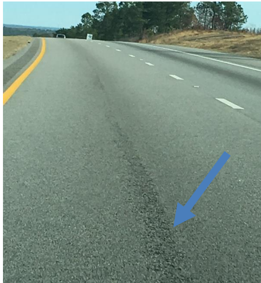
Figure 2.3- Raveling of OGFC on I-20 in Lugoff, SC
