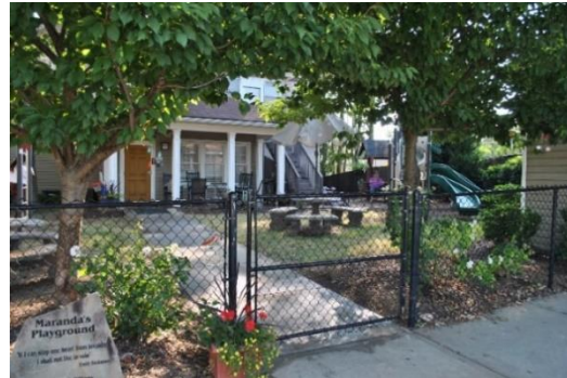
Figure 5.7. Pedestrian security gate
