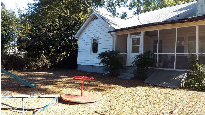
Figure 5.16. Exterior of shelter 2
