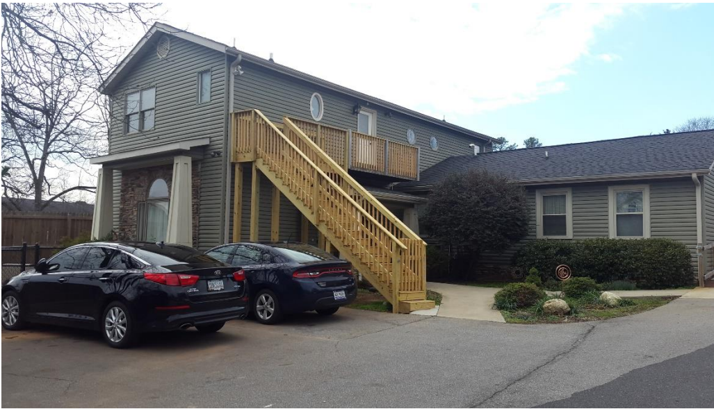
Figure 5.27. Exterior view of Site 3
