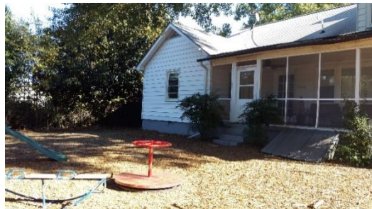
Figure 5.26. Screened porch looking over the play area
