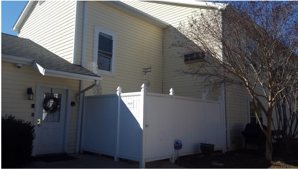
Figure 5.39. Exterior view of Site 4
