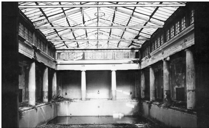
Figure 4.31: Interior of swimming pool building, 1970 (Lyndhurst Archives).
