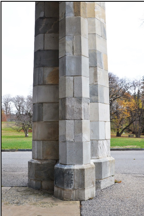
Figure 4.15: West side of south porte-cochère column (Photo by author).
