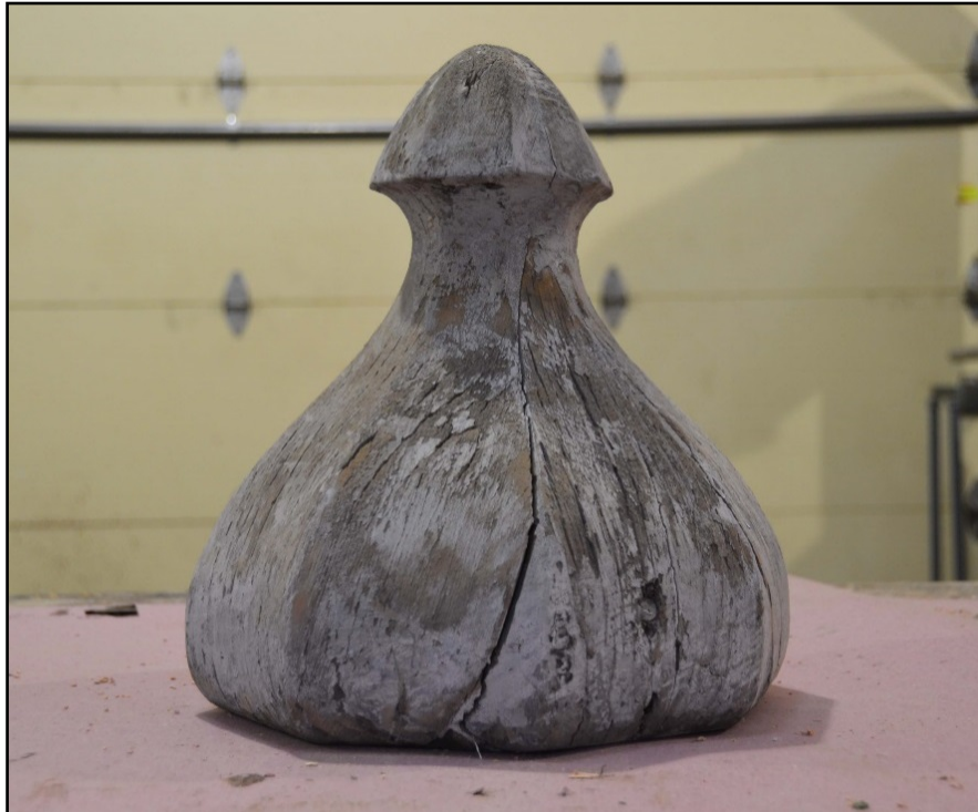
Figure 4.25: Original mansion roof finial (Photograph by author).
