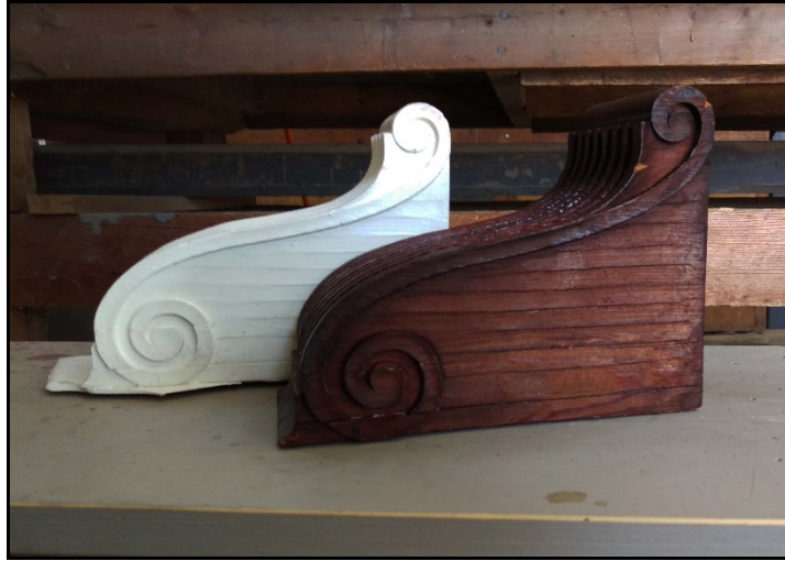
Figure 4.42: Small brackets, casting in white (Photo by author).
