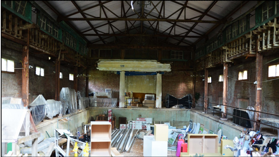
Figure 4.33: Interior of swimming pool building, 2016 (Photograph by author).
