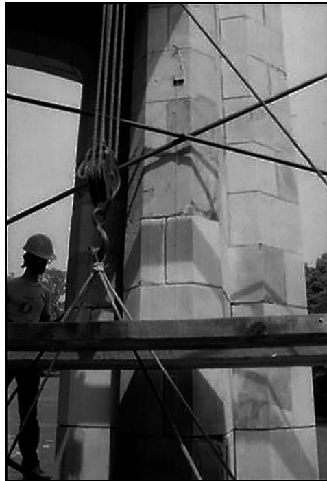
Figure 4.13: Installation of concrete (Lyndhurst Archives).
