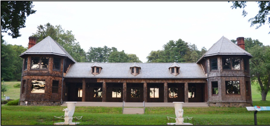
Figure 4.36: West elevation of swimming pool building, 2016 (Photograph by author).
