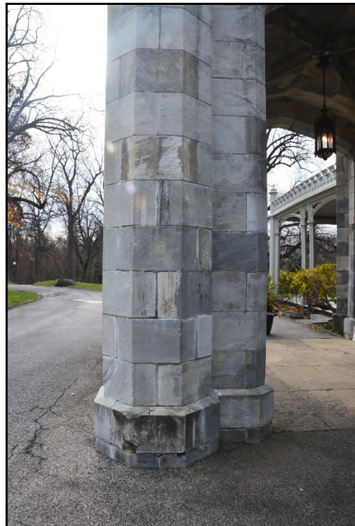
Figure 4.16: North side of south porte-cochère column (Photo by author).
