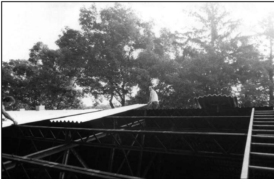
Figure 4.32: Corrugated aluminum roofing installation, 1984 (Lyndhurst Archives).
