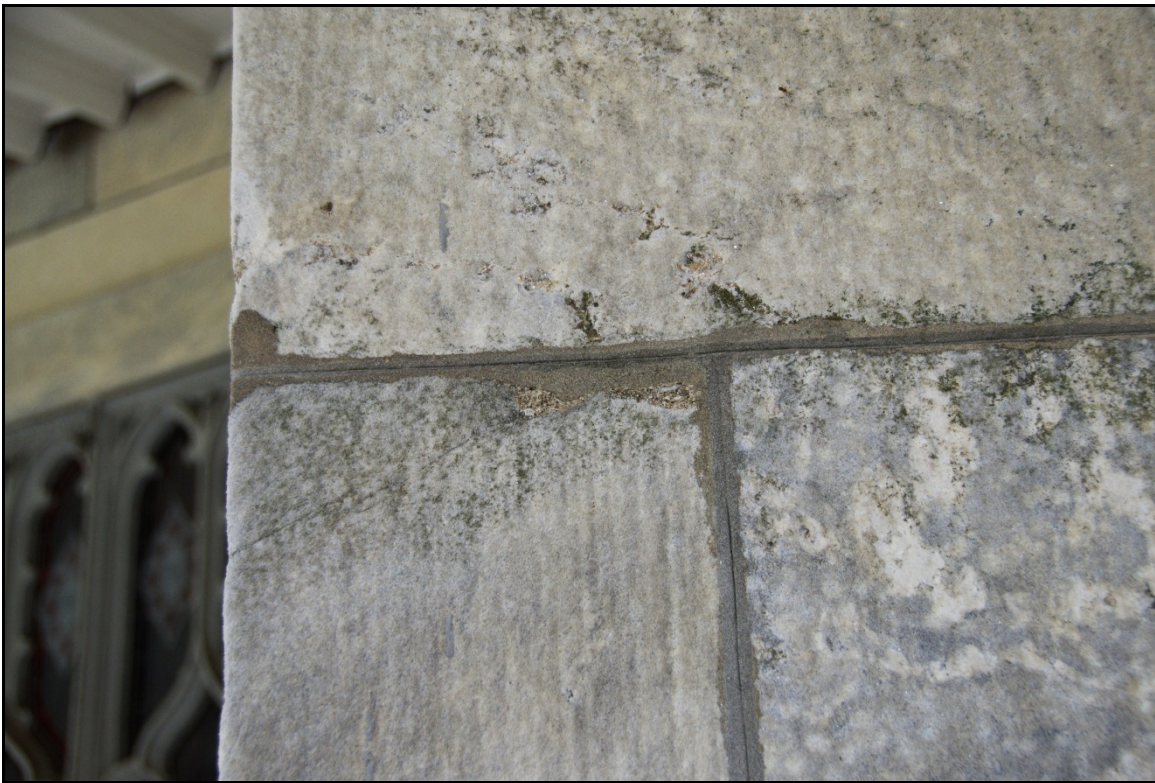
Figure 4. 6: Portland cement with surrounding patching of material loss and biological growth (Photograph by author).
