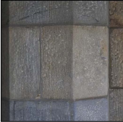
Figure 4.3: Original mortar (Photograph by author).
