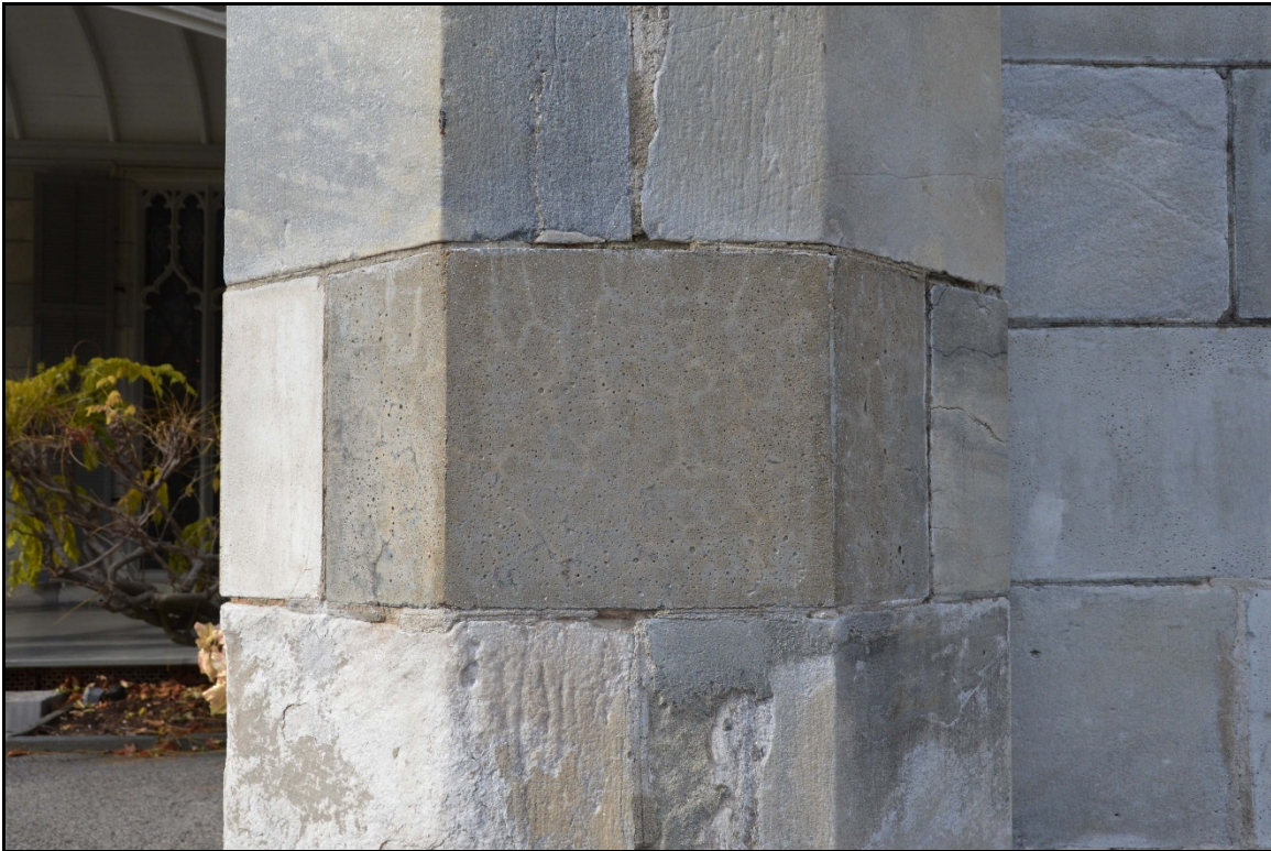
Figure 4.17: Detail of cast concrete and surrounding marble (Photo by author).
