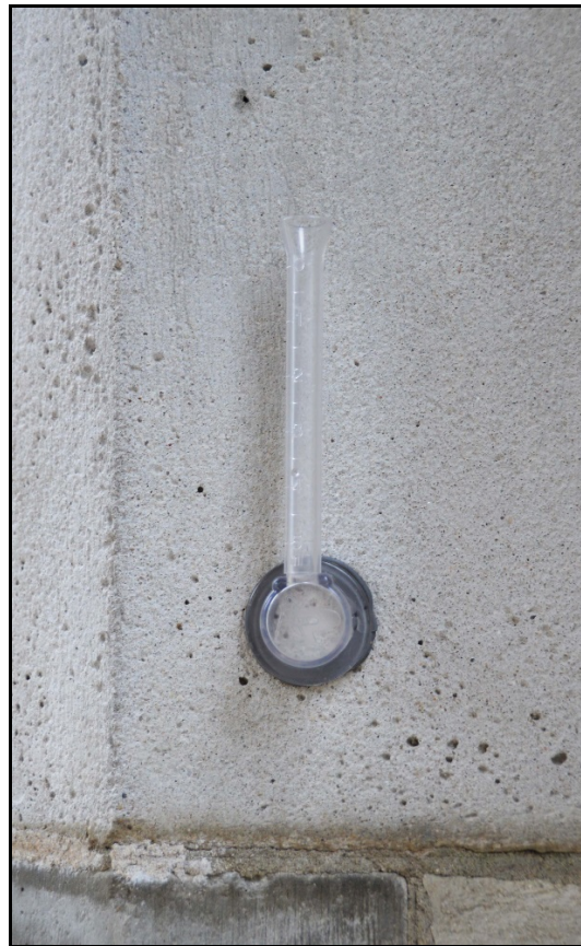
Figure 4.21: RILEM permeability testing of concrete (Photograph by author).
