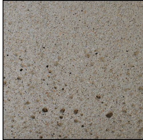
Figure 4.19: Detail of concrete texture (Photograph by author).
