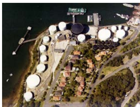
Figure 6. The BP Site in Waverton, in 1991, before demolition. (Photo courtesy NSW Lands Department)
