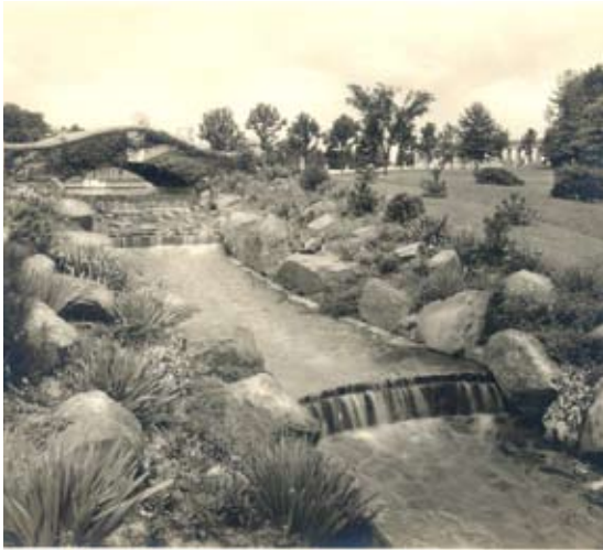
Figure 7. Masonry pond edges at Nemours. (Courtesy of Nemours Mansion and Gardens)
