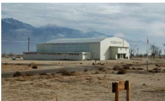
Figure 4. The auditorium from the northwest. The structure was in good condition when the NPS rehabilitated it into the National Historic Site's interpretive center. (Photo by author)
