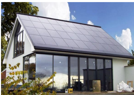
Figure 8: An in-roof system installation on a pitched roof
