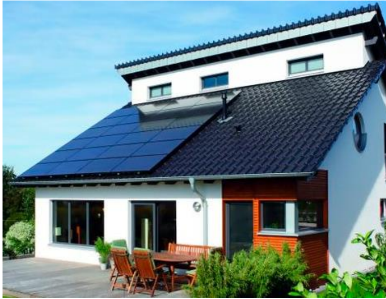
Figure 7: An erected system installation on a pitched roof
