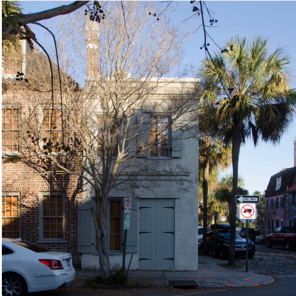
Figure 5.36 - Rectified Photograph for Measurement Purposes.
