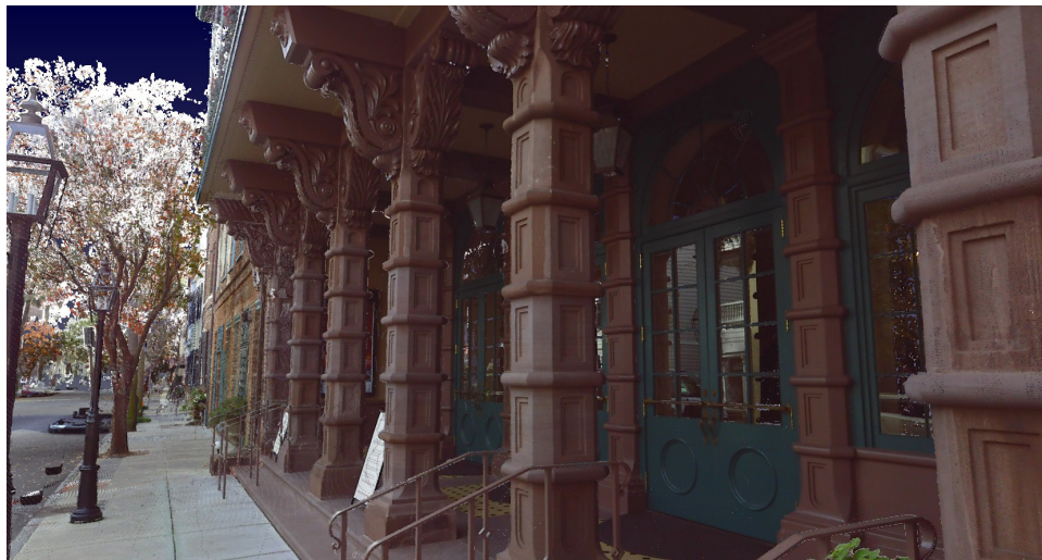
Figure C.6 - Laser Scan Detail of the Dock Street Theatre Portico.
