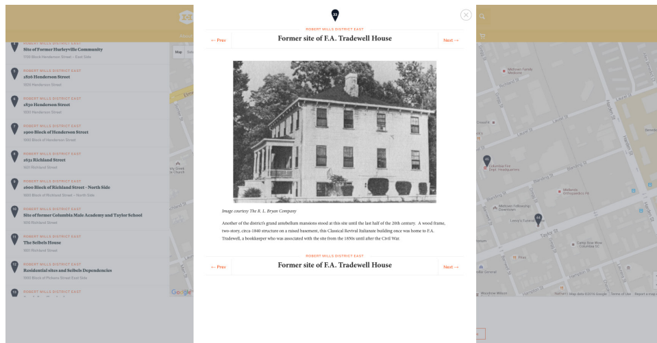
Figure 4.15 - F.A. Tradewell House in the Robert Mills District East.
