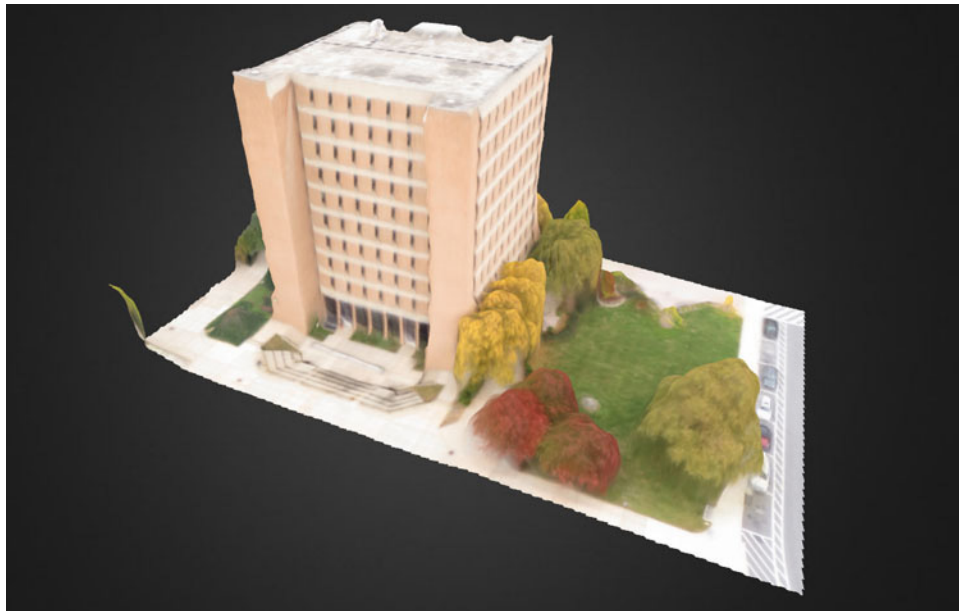
Figure 4.10 - UMBC Administration Building.
