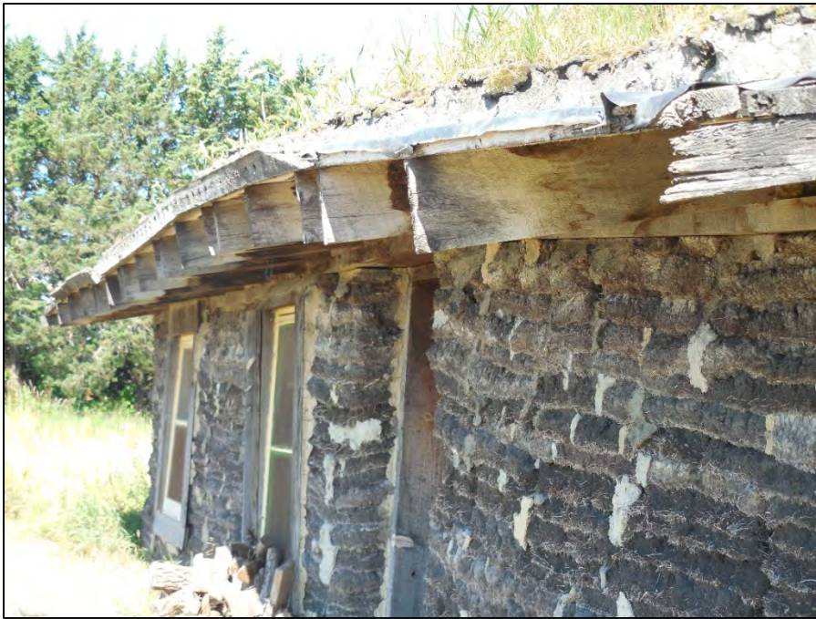
Figure 5.8: Sod House side view of roof
