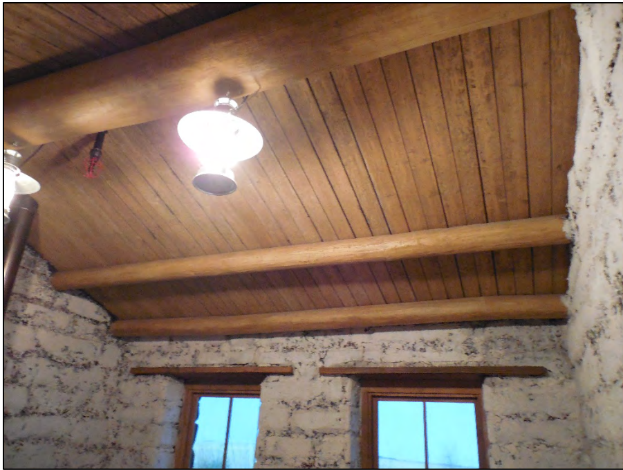
Figure 5.23: Interior roof finish
