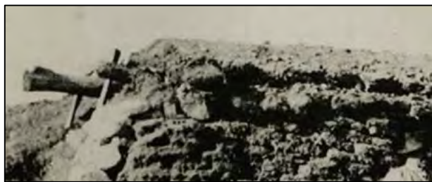
Figure 4.2: Sod Bricks and Logs Roof Example (Kansas Memory, Kansas Historical Society, 209059)
