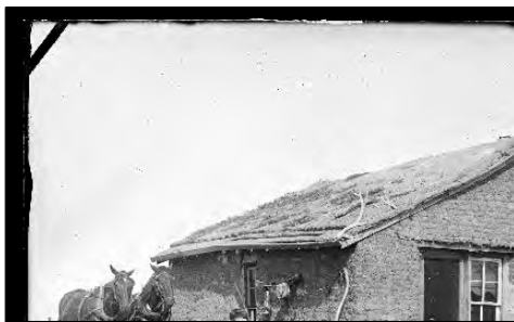
Figure 4.1: Sod Bricks and Lumber Roof Example (Nebraska State Historical Society [Digital ID nbhips 11019])
