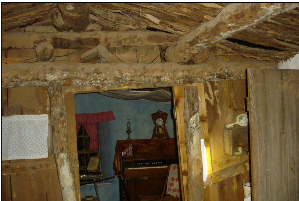
Figure 5.4: Interior Wooden Partition and Support Ridge Poles (Oklahoma Historical Society)
