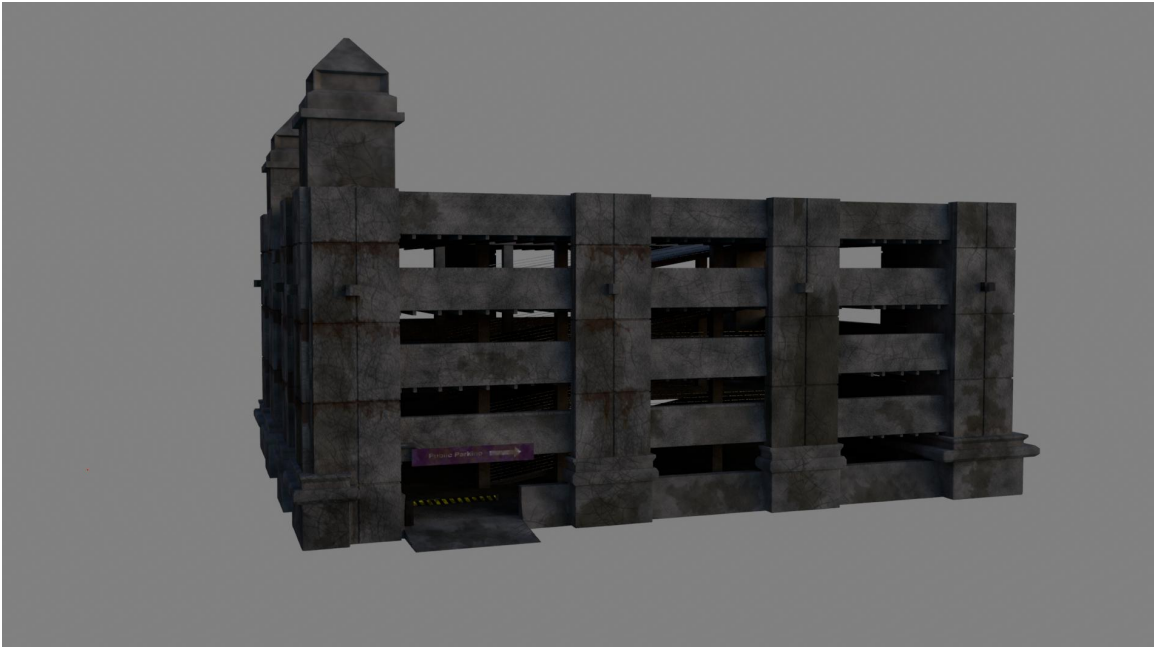
Figure 2.12: Parking Deck Surface
