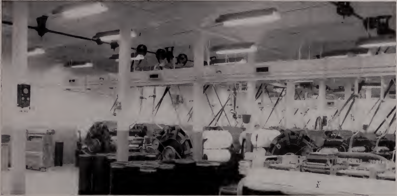
Card room at Highland Park Mfg. Co., Mill No. 1, Charlotte, N. C. Ductwork and zone central atomizers are part of Amco's central station system, designed by J. E. Serrine Company for the entire mill.
