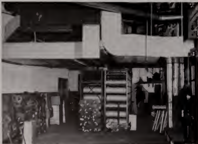
AMCO Unit Dry-Duct System at The Windsar Manufacturing Company, Philadelphia, Pa. The entire unit is installed overhead out of the way.
