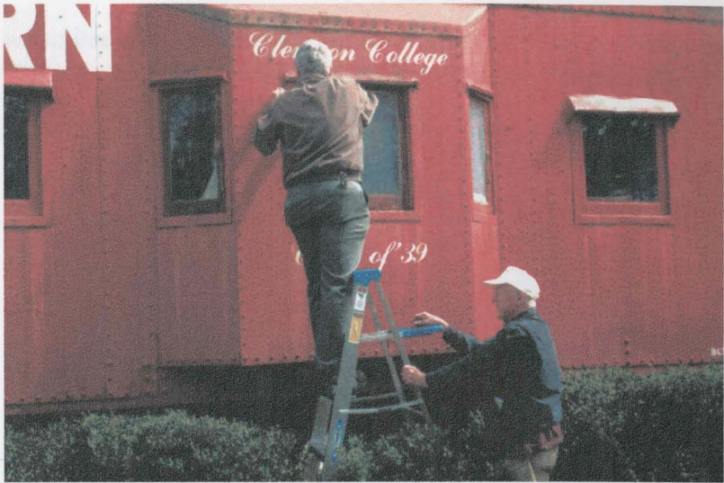
Tee supervises (?) Bud Bodine's installation of a new window
