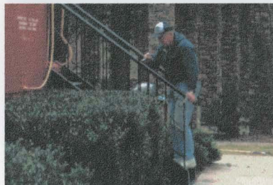
Ray Turner does a final touch-up on the steps
