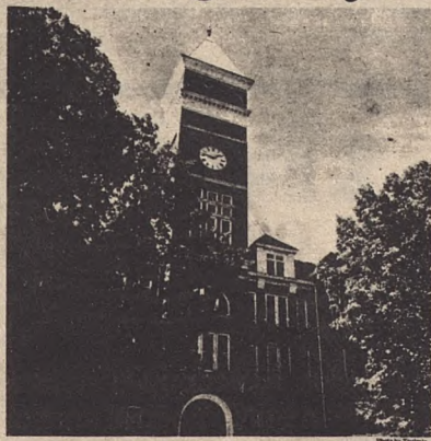
renovation of Tillman "must meet all requirements for the handicapped and, in addition, it must meet new safety standards."
