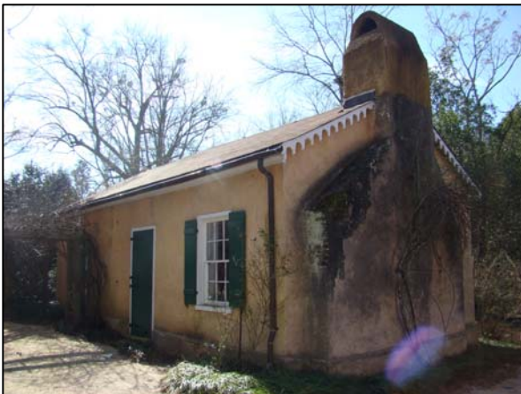
Figure 78. The east façade of the dairy/kitchen building. (Photo: Author)
