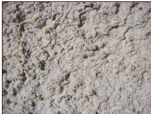
Figure 134. View of the current cementitious exterior pebble dash render. (Photo: Author)
