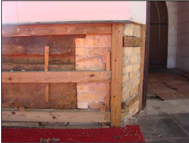
Plate A21. Brick repair made near the porch entrance on the south elevation. (Photo: Author)
