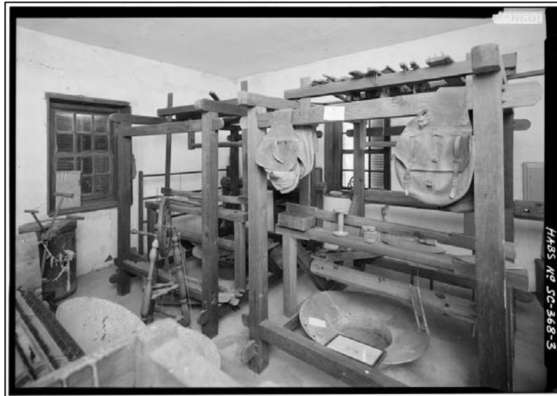
Plate A7. Interior of the loomhouse showing the looms that are currently in poor condition. (Photo: Library of Congress)
