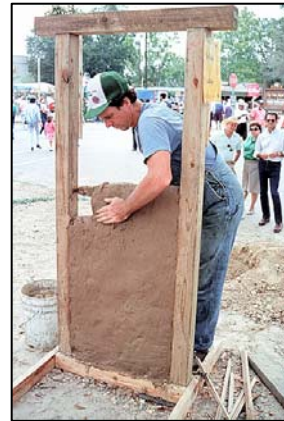
Figure 21. A man demonstrating how a bousillage wall is made. (Photo: www.laheritage.org )
