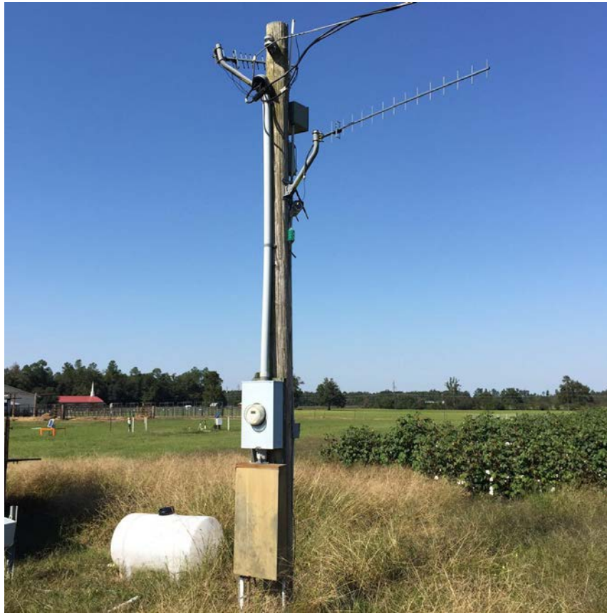
Figure 1.18 Gateway antennas nearby the test field.
