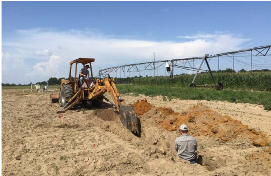
Figure 1.5 Digging trench for sensor calibration.
