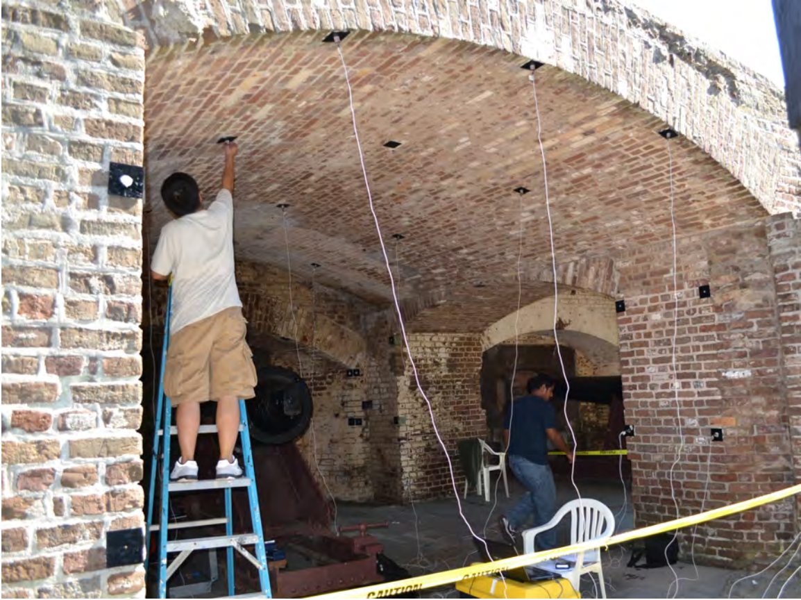
Figure 31: The experimental set-up showing accelerometers mounted on the vaults and piers.
