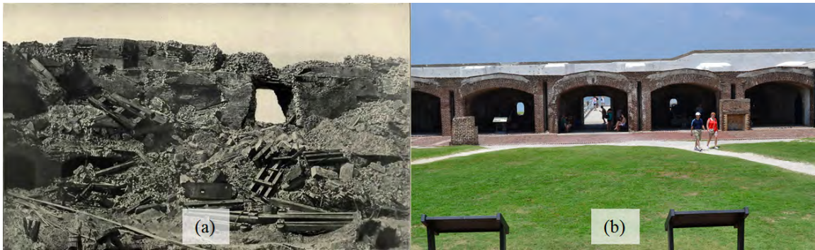
Figure 25: (a) Photo taken on August, 1863 showing the first breach in Fort Sumter walls (original photograph by G.S. Cook), (b) Photo taken in August, 2011 showing the current condition of Fort Sumter casemates.
