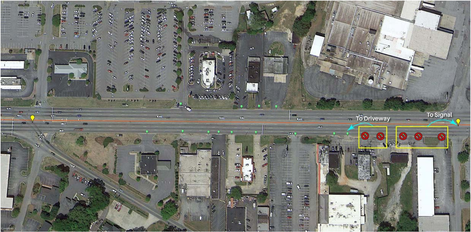
Figure 13b – Closing of Driveways within Minimum Acceptable Corner Clearance along Wade Hampton Blvd (cont. on following pages).
