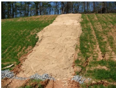
Test bed location (left)
