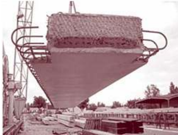
Figure 2.5: Poutre Dalle System (Ralls et al. 2005)
