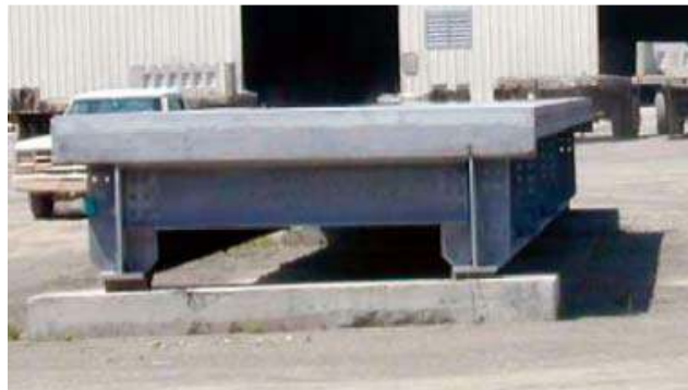
Figure 2.20: Inverset System Unit (New York) (Culmo 2009)
