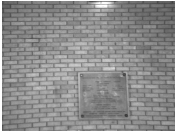
Figure 4.2 Right Image Brick Wall
