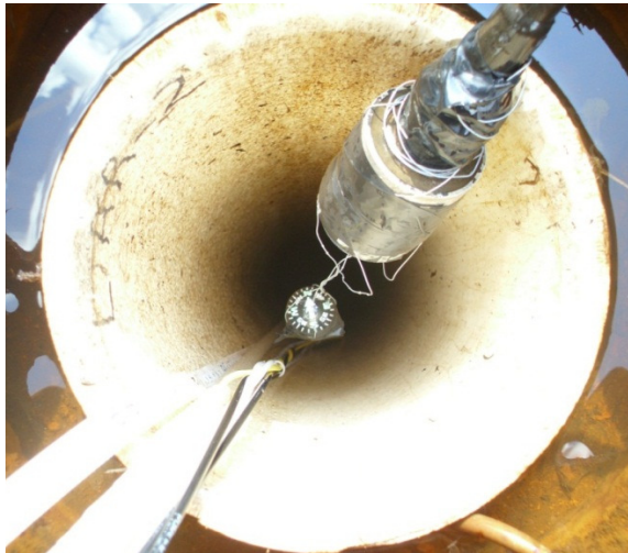
Figure 3.10: The compass used to determine the orientation of the 3DX in the borehole before a well test. The resolution that can be seen using the camera and compass set up is approximately \pm 20 degrees.
