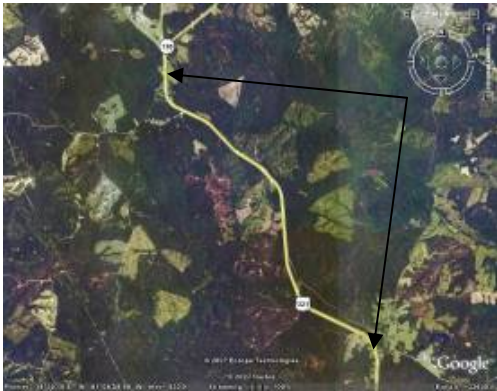
Figure12: SCDOT Test Road*
