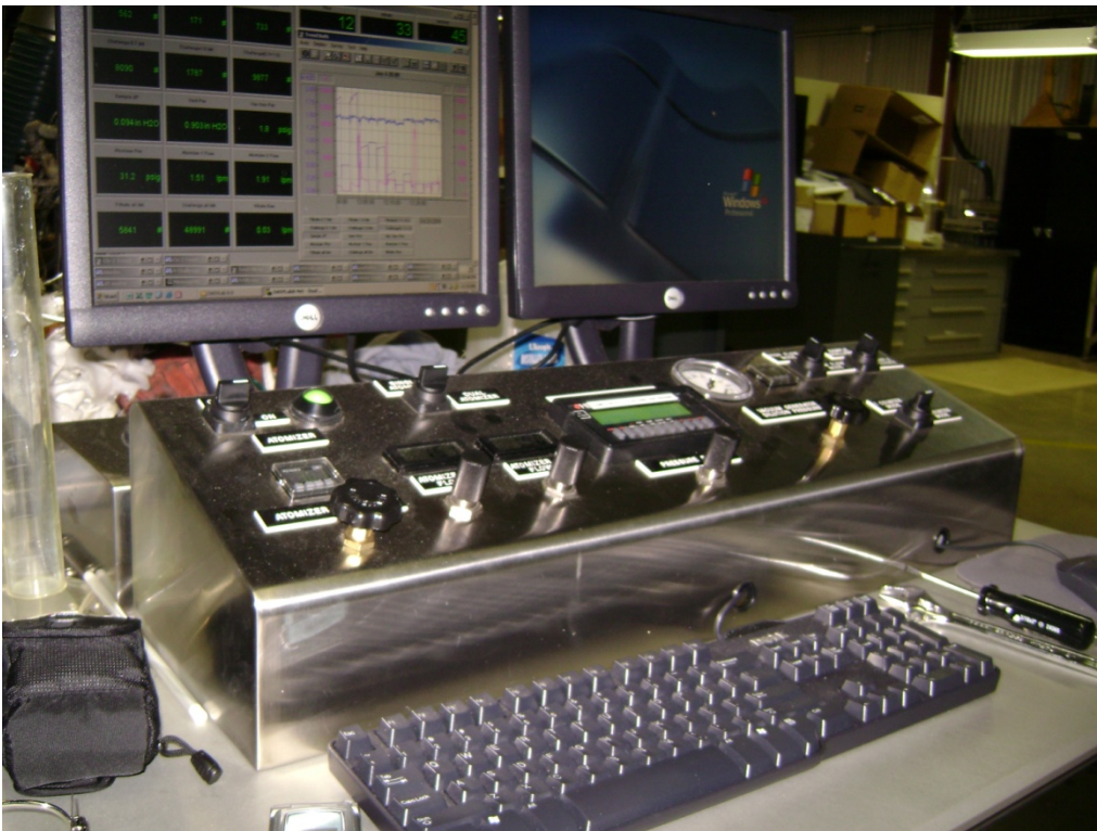
Figure 20: System control panel
