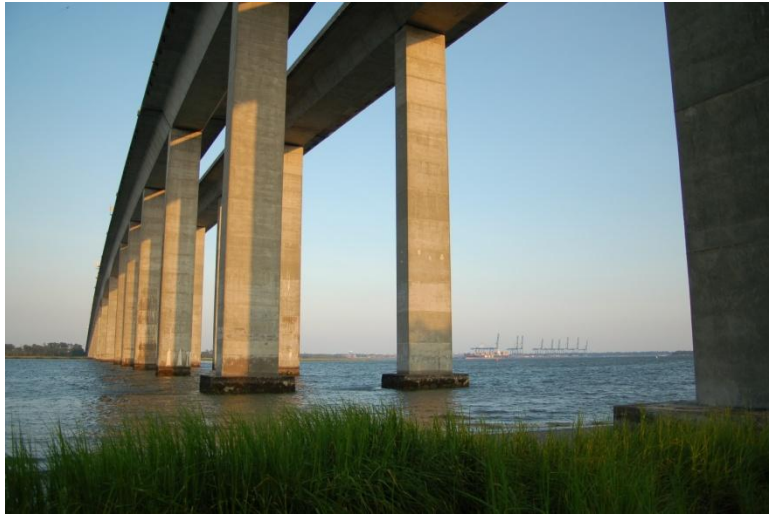
Figure C-2. James B. Edwards Bridge over Wando River
