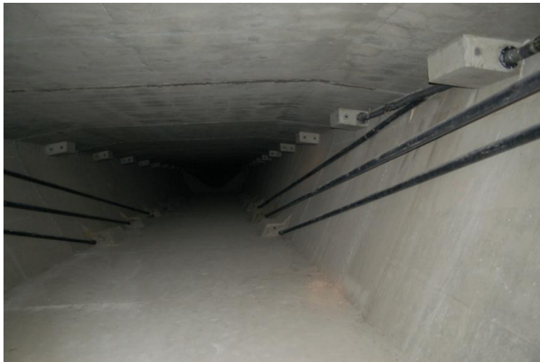
Figure C-3. View Inside James B. Edwards Bridge
