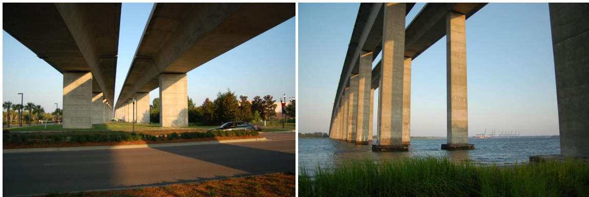
Figure 3-3. James B. Edwards Bridge of Charleston, SC
