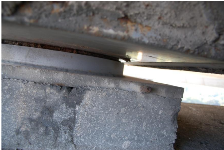
Figure C-8. James B. Edwards Bridge Bearing
