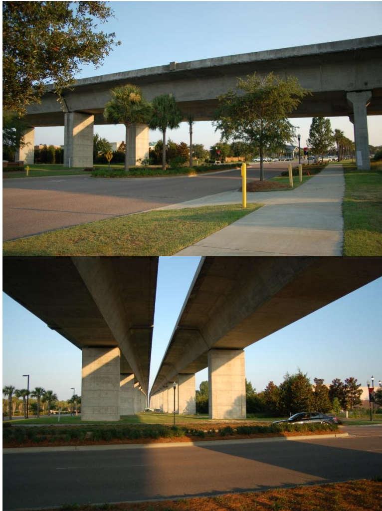
Figure C-1. Roadway beneath James B. Edwards Bridge
