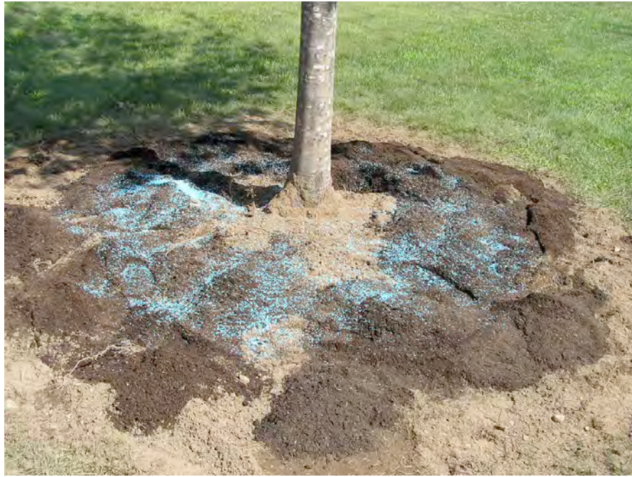
Figure 6.1. Soil beneath red maple tilled with Airspade ® and amended with fertilizer and compost before (incorporation into soil profile).
