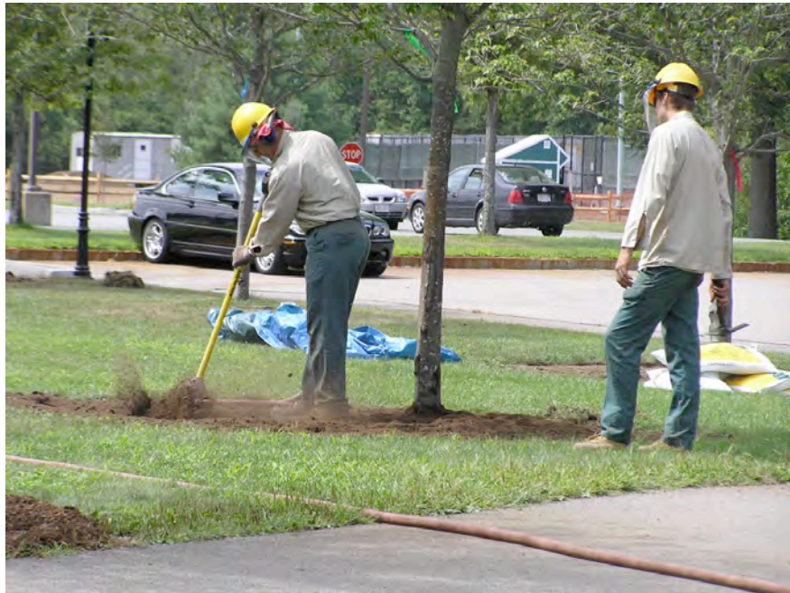
Figure 6.2. Incorporation of amendments into the soil profile using the Airspade ® .
