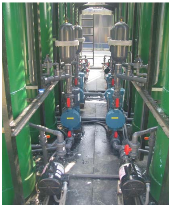
Figure 11: Ammonia Recovery Process at "landfill site II", showing green absorption columns and acid spray pumps.
