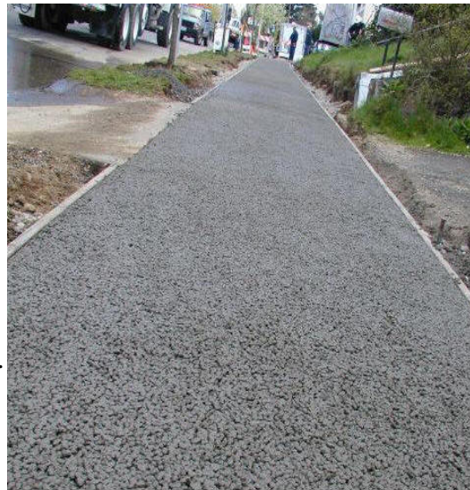
Figure 2.4: Pervious concrete roadway
