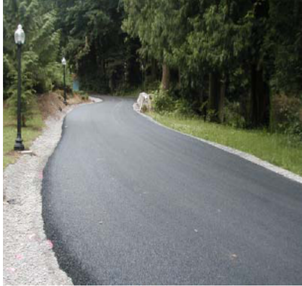
Figure 2.5: Porous asphalt Source: Lake Superior Streams, (2007)
