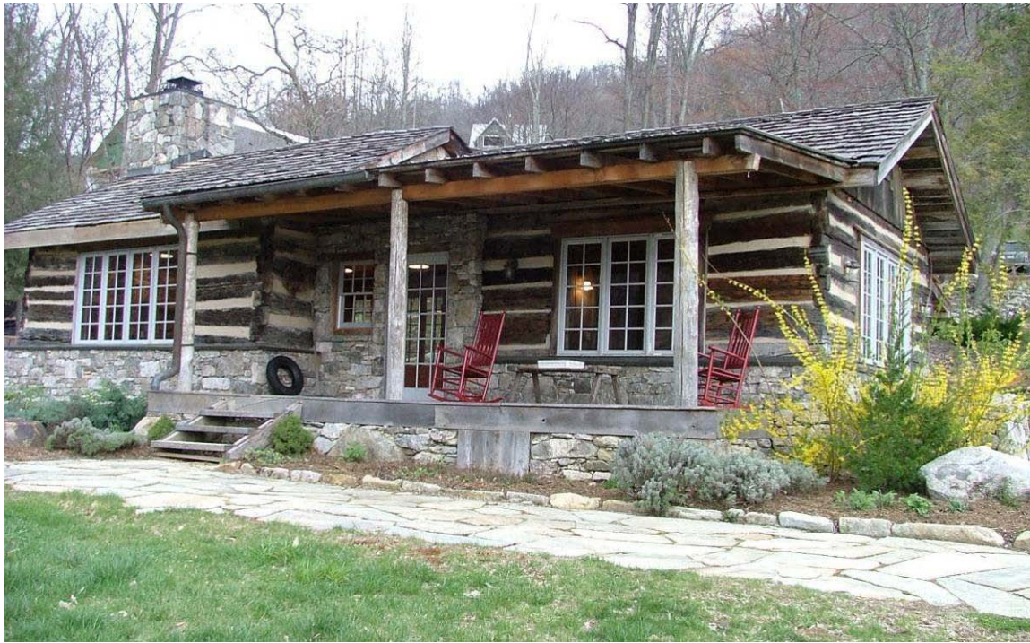
Figure 8.37: “Homestead Cabin” incorporates parts of a 1800s hewn log chapel (Source: Author).
