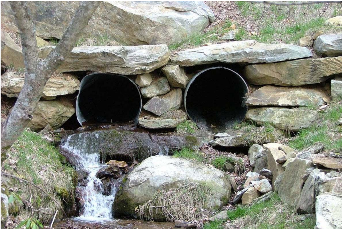
Figure 8.24: Culverts on the stream (Source: Author).
