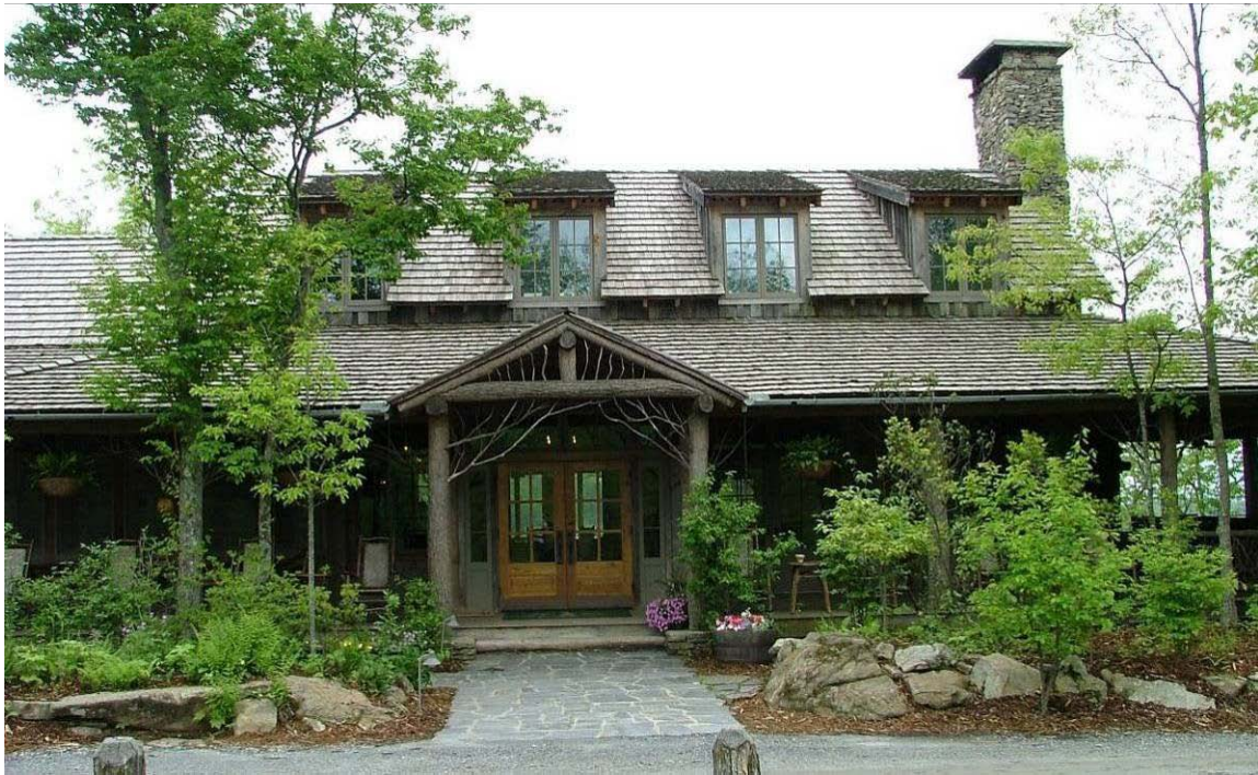
Figure 5.34: The Boarding House at Balsam Mountain Preserve (Source: Author).
