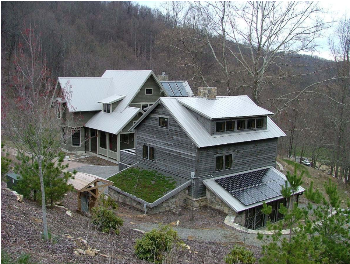
Figure 8.39: Solar panels and a green roof adorn the 2008 Southern Living farmhouse (Source: Author).
