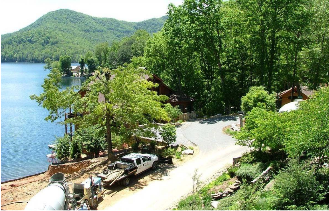
Figure 7.48: Site preparation for lakefront home (Source: Author).
