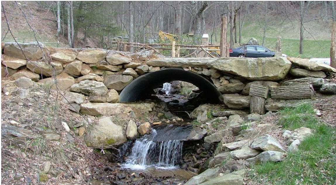
Figure 8.23: A large half culvert allows the existing stream channel to remain intact (Source: Author).
