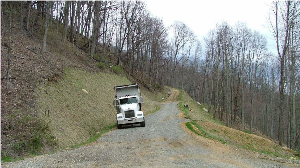
Figure 8.26: Steep topography found on site necessitates substantial grading for road placement (Source: Author).
