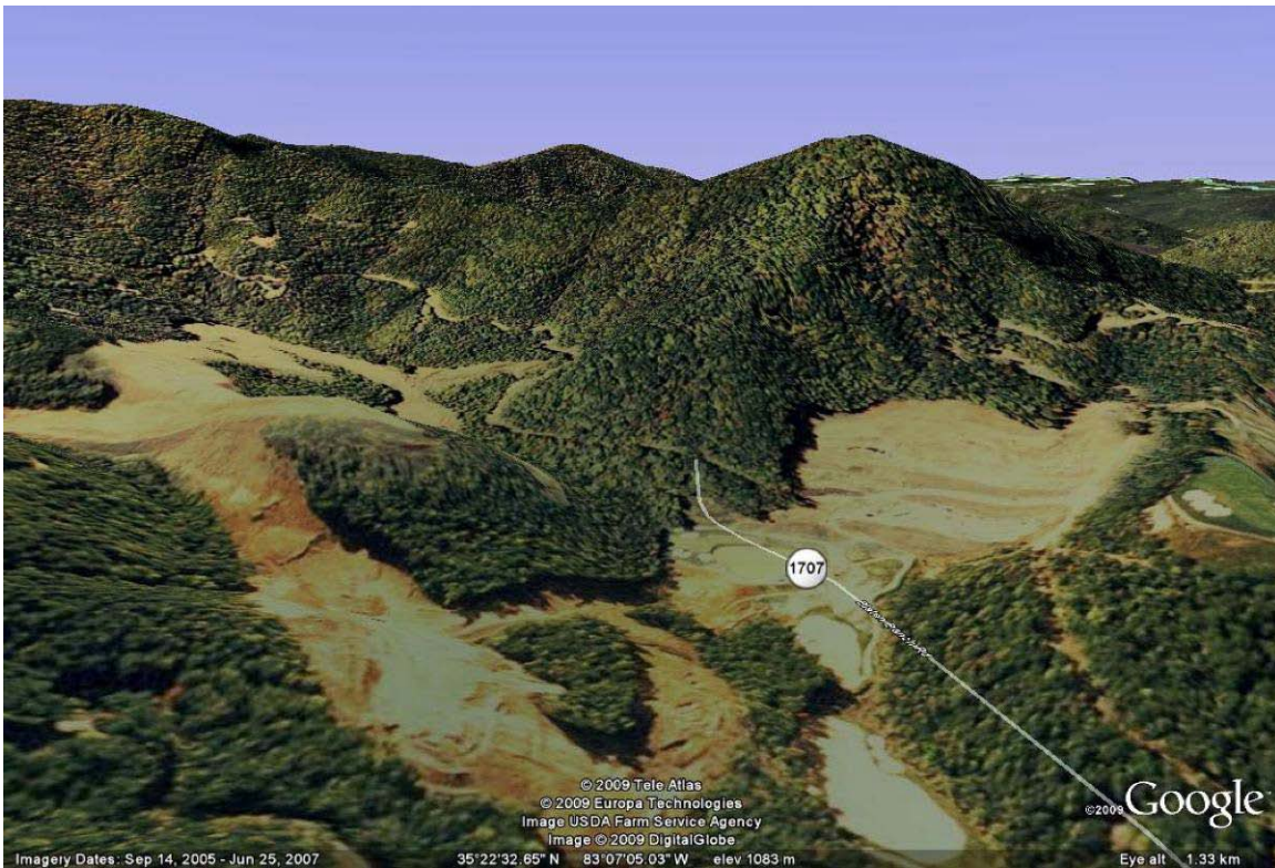
Figure 9.3: Construction of Balsam Mountain Preserve’s golf course captured by Google Earth (Source: Google Earth, 2009).
