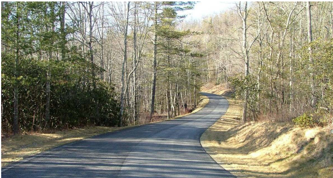
Figure 6.29: Typical access road in Chinquapin (source: Author).
