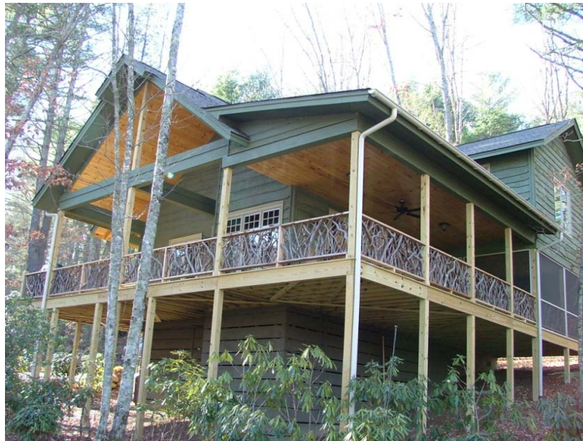
Figure 2.1: Architectural detailing and color palette help a newer home to blend into its surroundings (source: Author).
