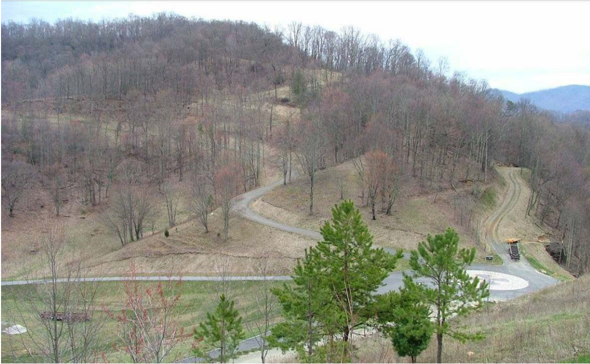
Figure 8.25: Access roads throughout the project (Source: Author).
