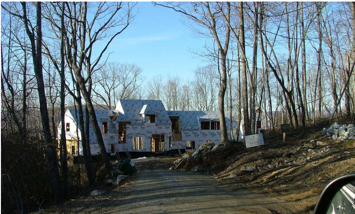
Figure 6.49: New home undergoing construction (source: Author).
