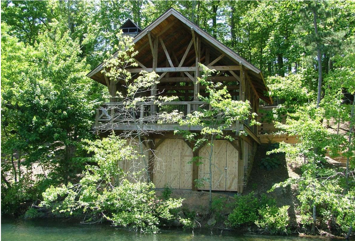
Figure 7.34: Santeetlah Lakeside pavilion (Source: Author).
