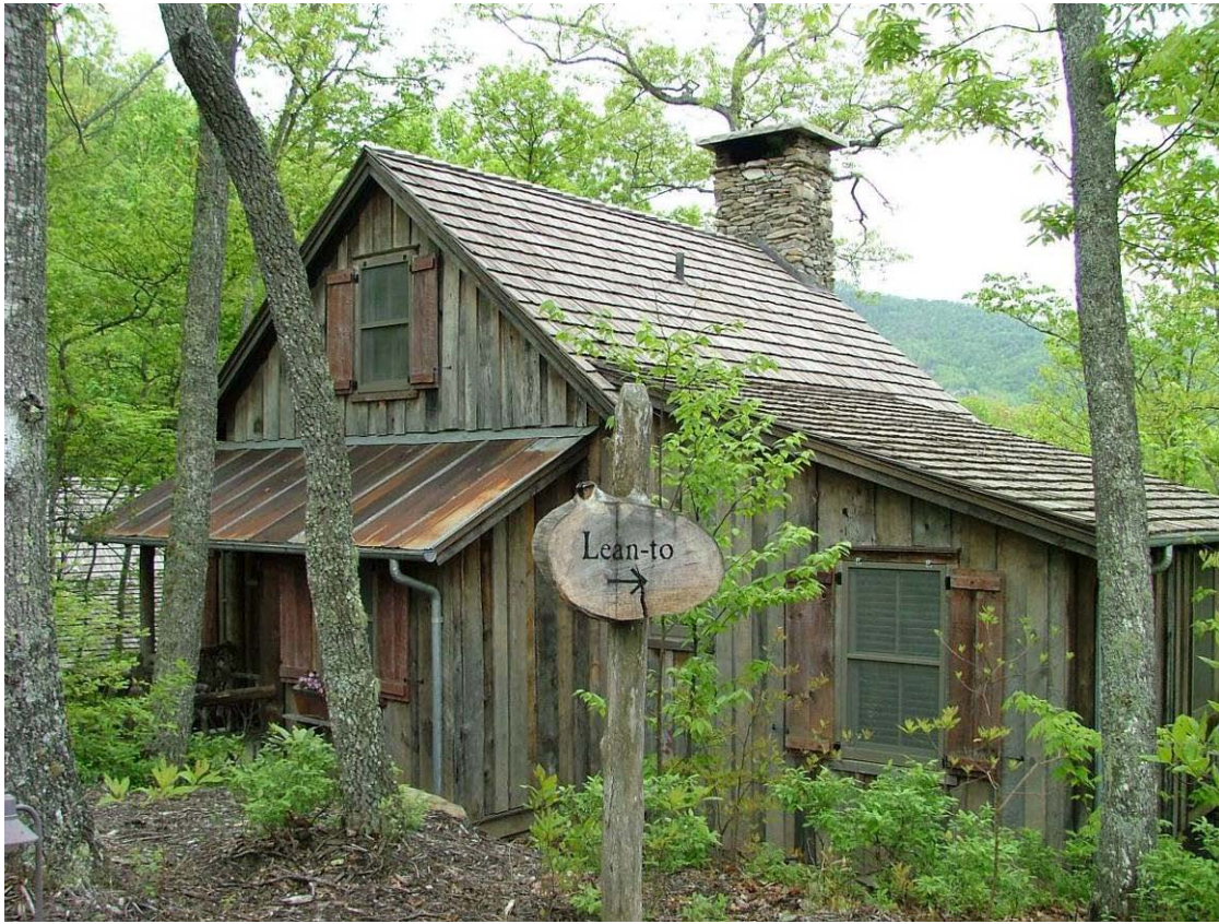
Figure 5.38: Boarding House Cabins offer fractional ownership (Source: Author).
