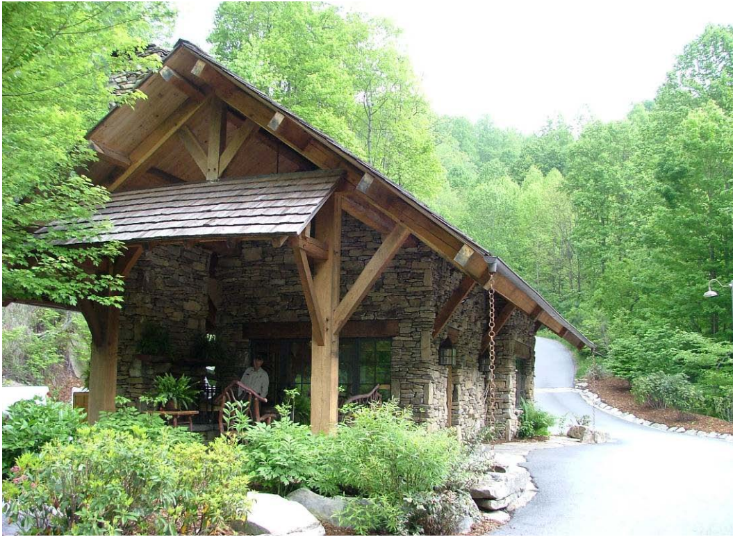
Figure 5.23: Balsam Mountain Preserve guard house (Source: Author).
