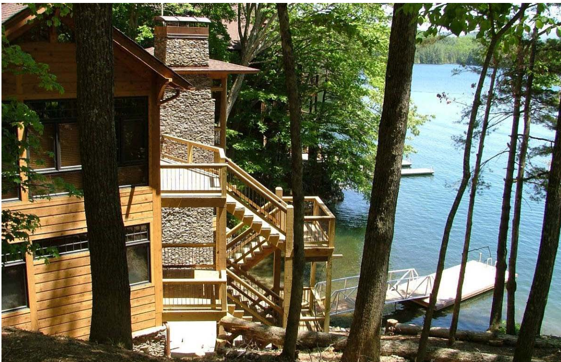
Figure 7.45: Lakefront home built directly on the shore (Source: Author).
