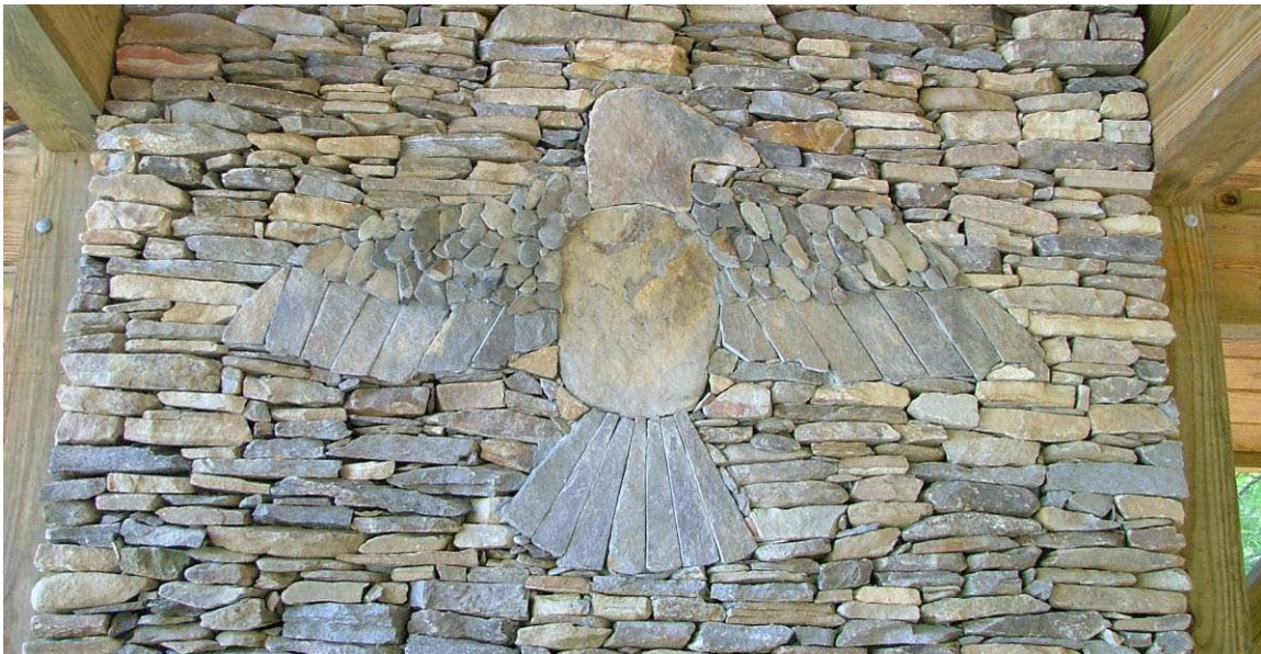
Figure 7.35: Stonework in lakeside pavilion chimney (Source: Author).
