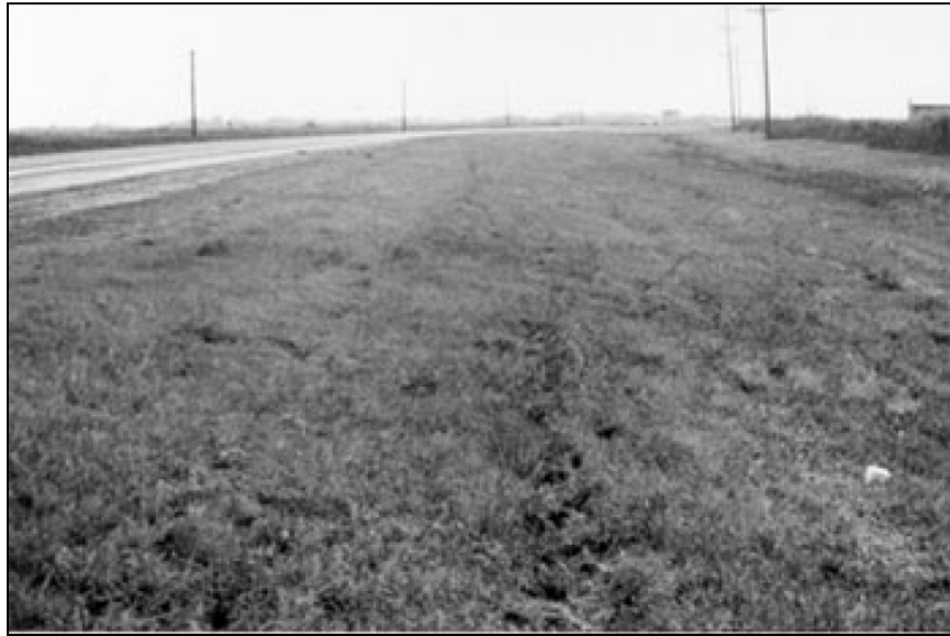
Clear zone greater than or equal to 30 ft sideslope flatter than 1V:4H, recoverable.
