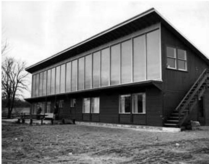
Figure 2.6: In the Dover house the solar panels with Glauber's salt sat directly behind a bank of eighteen windows that lined the second story of the south-facing wall. (Source: Sherburne, 2009)
