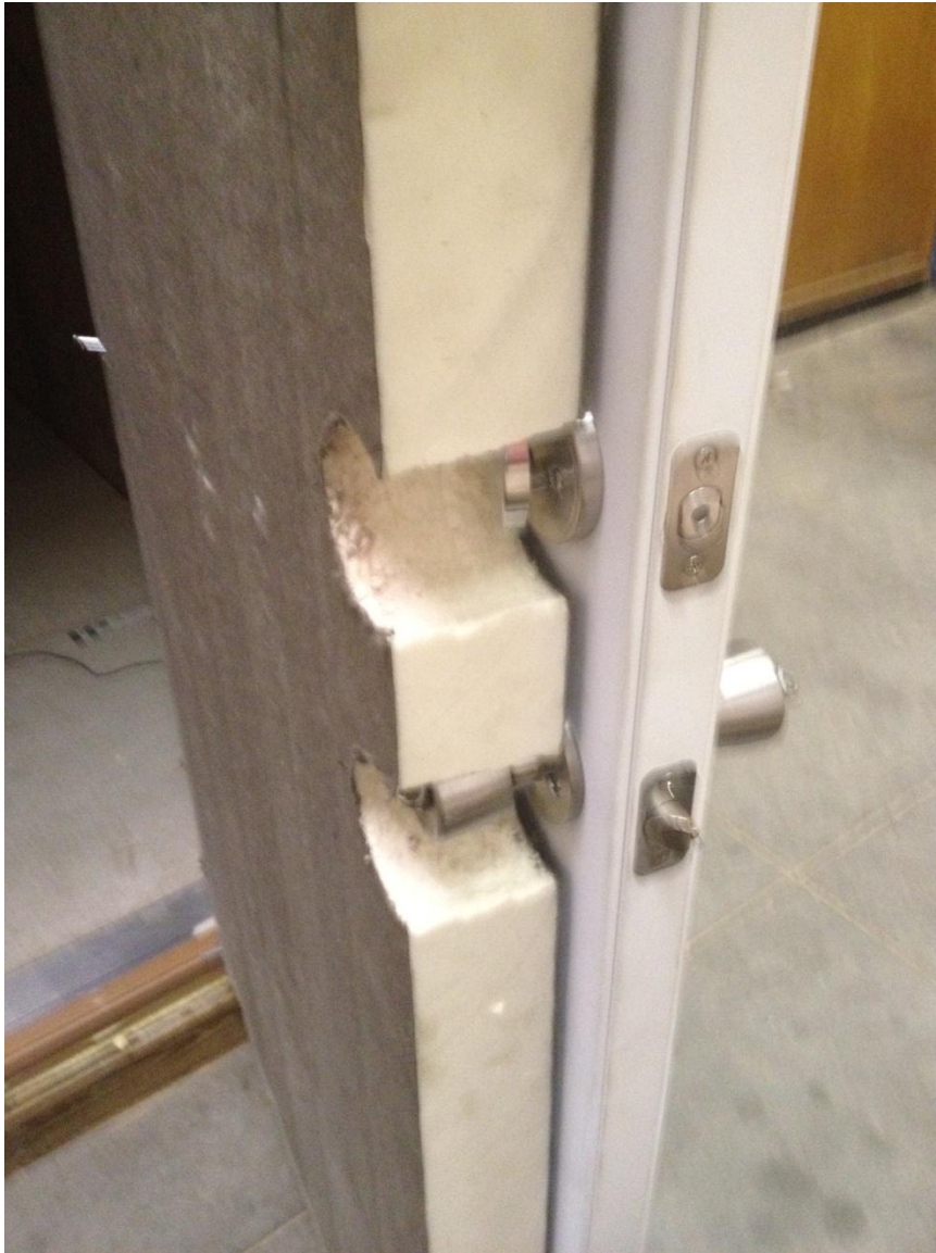
Figure 3-3: The insulation on the door to the experimental room
