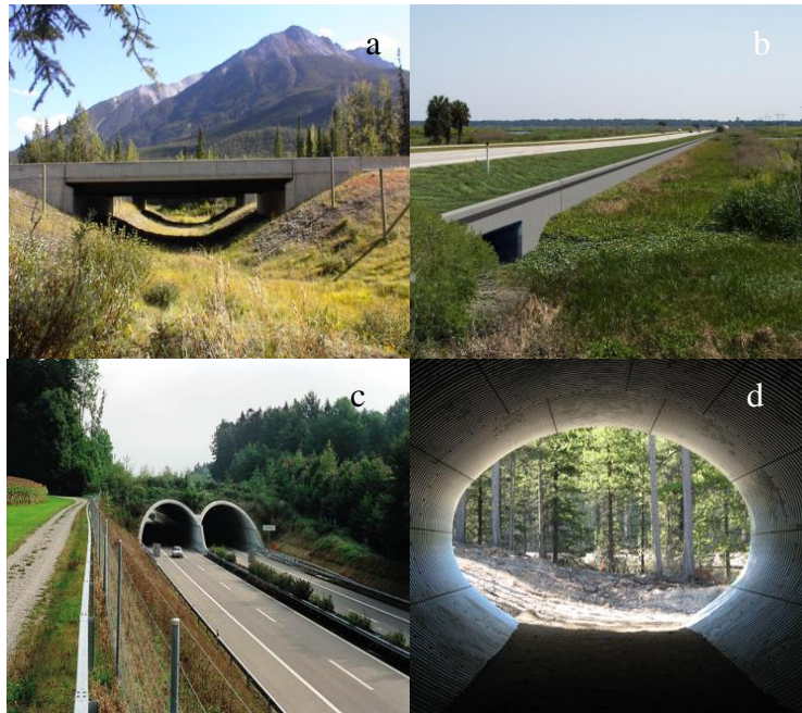
Figure 4.3: Samples of dedicated animal passages for roadways: (a) wildlife underpass (CPWS, 2012), (b) Payne prairie ecopassage (TLJE, 2012), (c) wildlife overpass (FHWA, 2012), and (d) wildlife culvert (Parks Canada, 2012)
