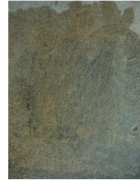
Concrete with wet sand
