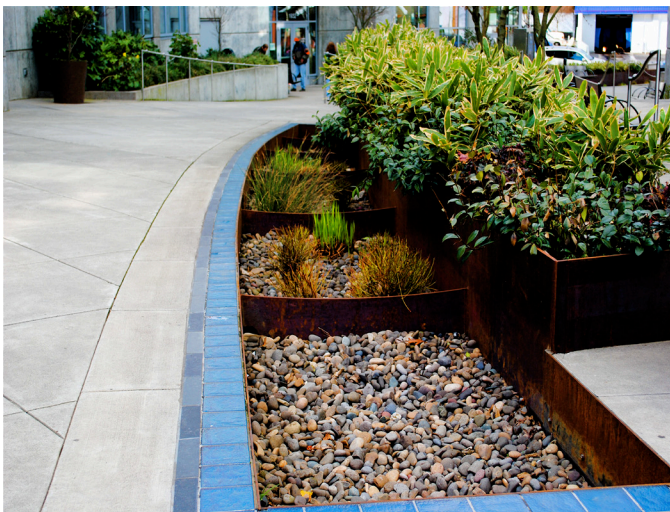
Picture 11: Rain Garden
