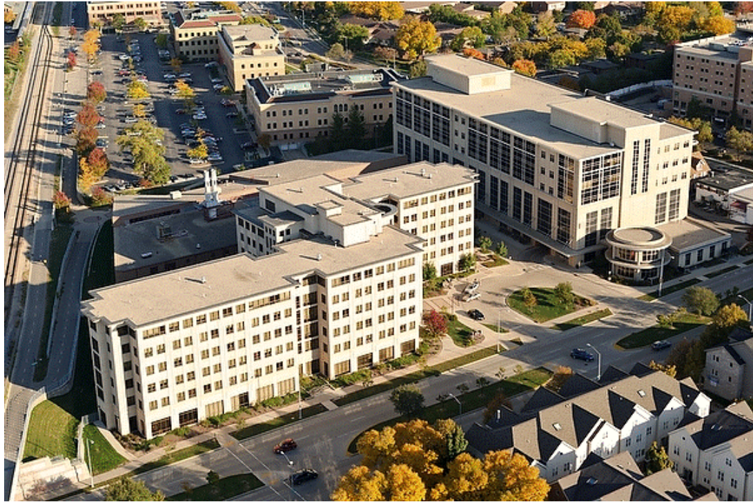
Figure 5.2: Photograph of Newell Smith Hall. Permission to use granted by the University of Wisconsin Madison.
